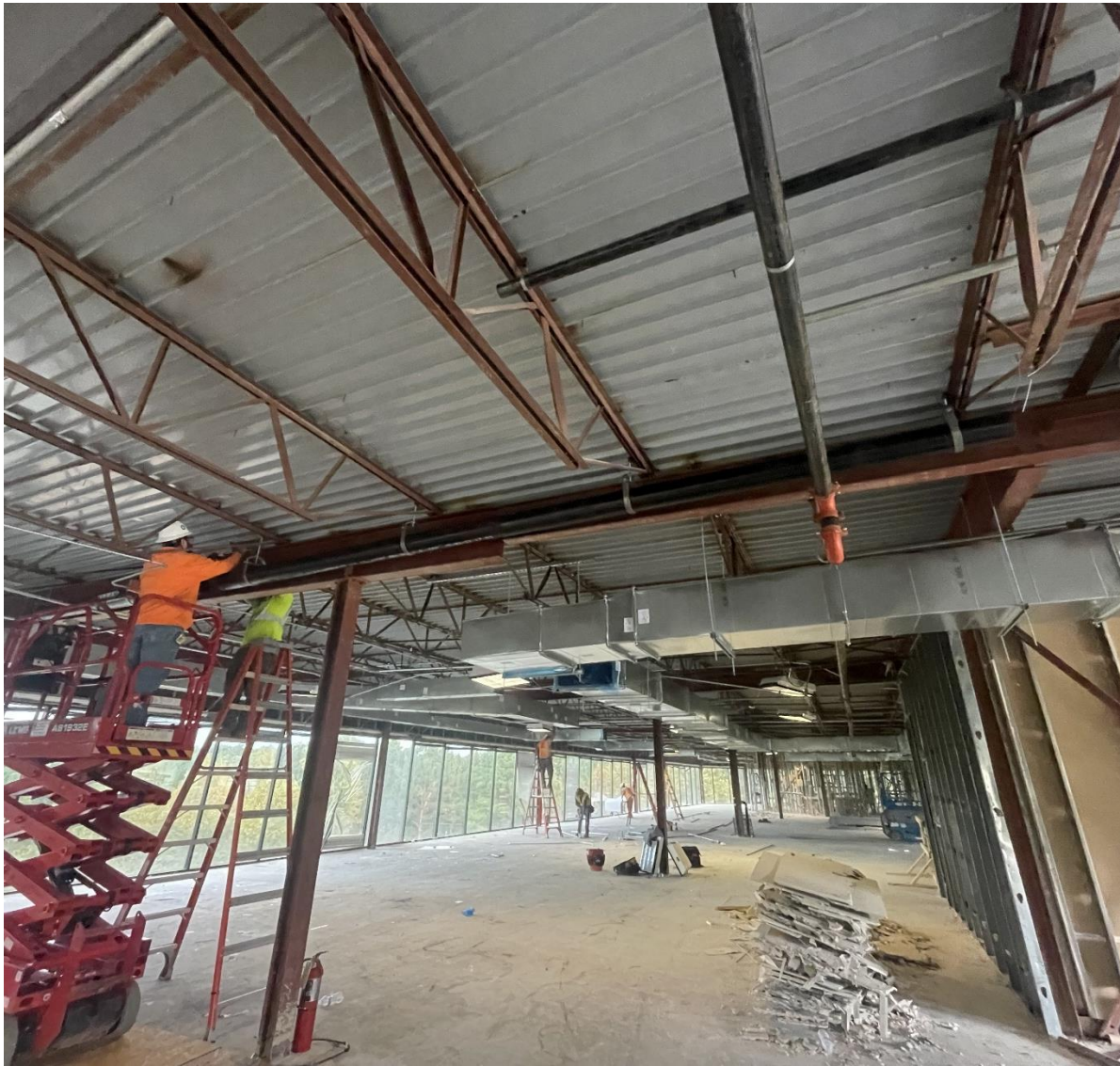
Continue Overhead MEP Rough-in On Level 3
