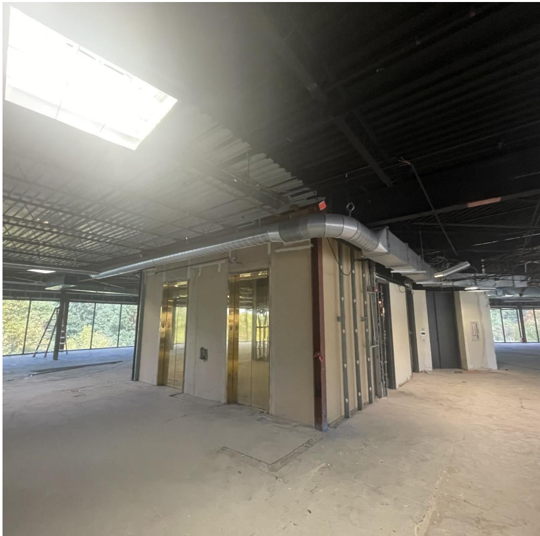
Begin Wall Layout On Level 3
