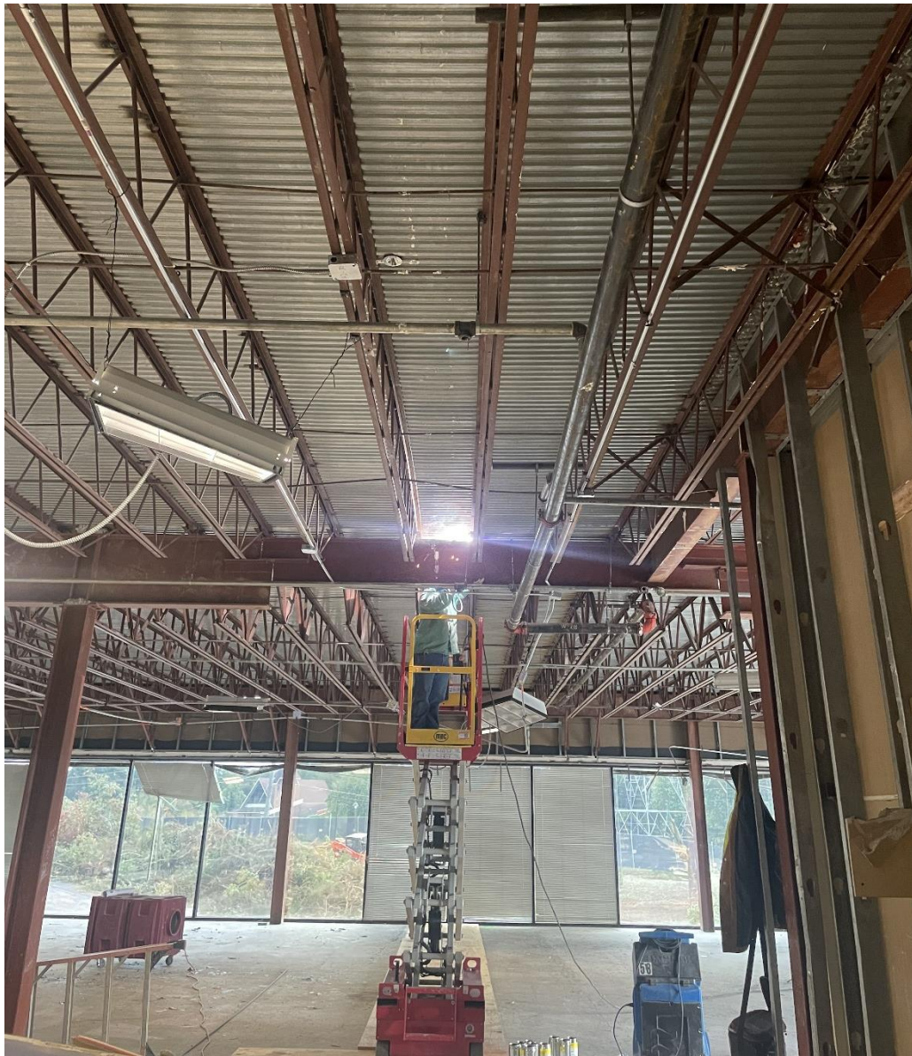
Continue Joist Augmentation On Level 2
