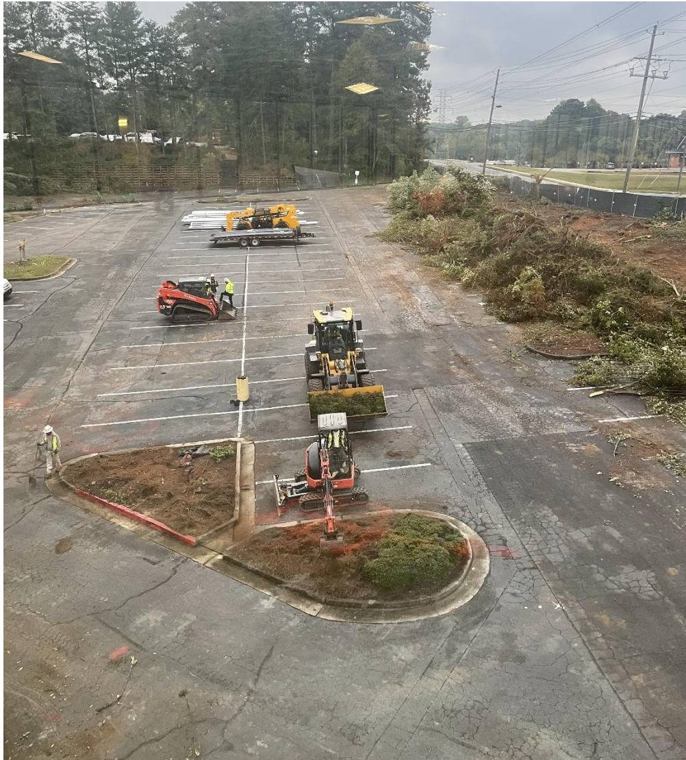
Clearing And Grubbing Of The Site
