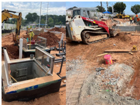
Photo Description (left to right): Vault ladders installed. Prepping foundation of middle basin, Completed pour of gap in Mt. Vernon Highway Wall
