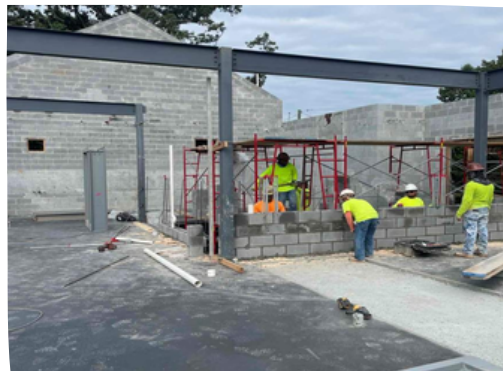
Photo Description (left to right): Elevated Slab on Deck Prep at the Second Floor, Continuing Installation of Interior CMU, Continuing in-wall Rough-in
