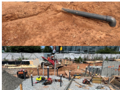
Photo Description (left to right): Completed flagpole installation/continued granite curb installation, Continued with underground fountain plumbing, Electrical Panel install & prep for conduit under Mt. Vernon Highway wall.
