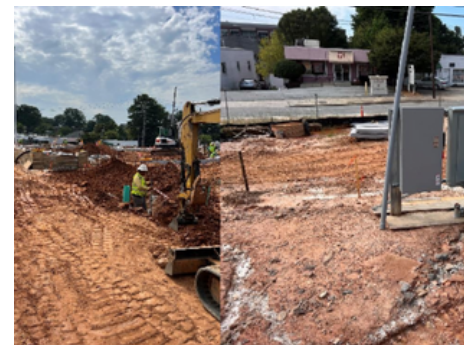
Photo Description (left to right): Completed flagpole installation/continued granite curb installation, Continued with underground fountain plumbing, Electrical Panel install & prep for conduit under Mt. Vernon Highway wall.
