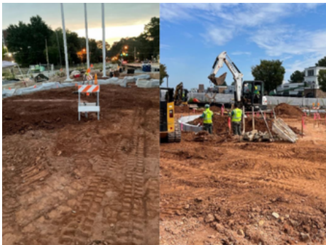
Photo Description (left to right): Completed flagpole installation/continued granite curb installation, Continued with underground fountain plumbing, Electrical Panel install & prep for conduit under Mt. Vernon Highway wall.
