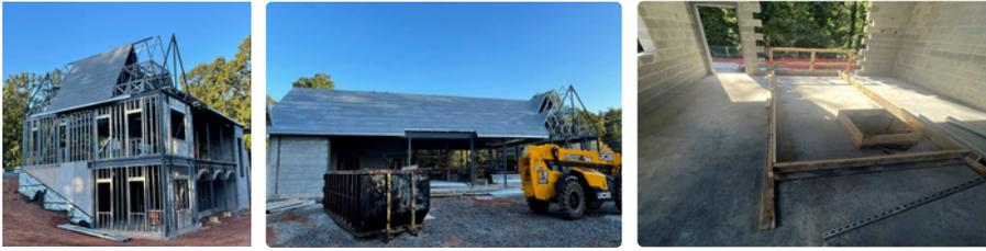
Photo Description (left to right): Continued Exterior Framing at the First and Second Floor, Continued Installation of Roof Decking, Formwork for Generator Pad at the Electrical Room
