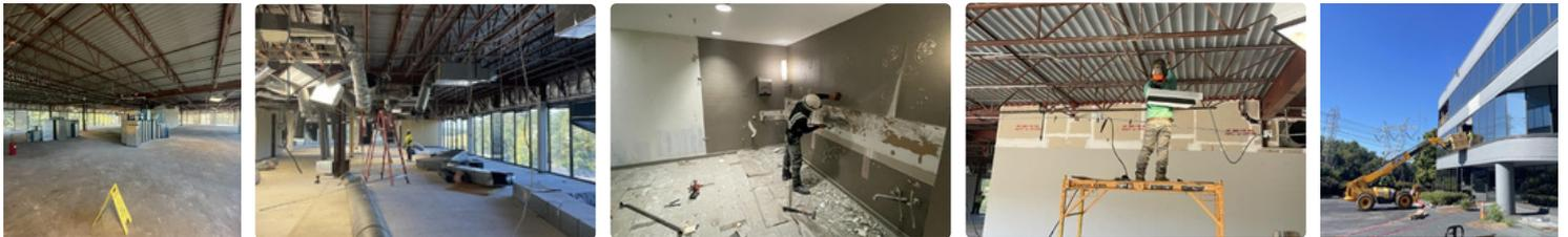
Photo Description (left to right): Staging Material for OH Mechanical Rough, Continue Demo of MEP overhead, Demo of Existing Conditions, Begin joist augmentation, Exporting Demo'd Material
