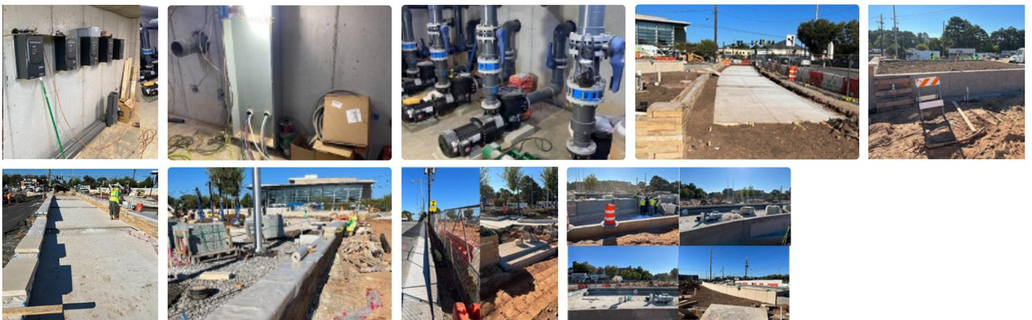
Photo Description: Top (left to right) - Continue install of equipment in vault (first three photos), Completed pour of northern section of Johnson Ferry sidewalk, Completed pour and soil of southern Roswell Road planter. Bottom (left to right) - Continued install of precast wall cap on JFR and Mt. Vernon (first two photos), Poured Roswell Rd. curb and planted trees in monument area, Continued installing tile and precast veneer finishes on fountain.
