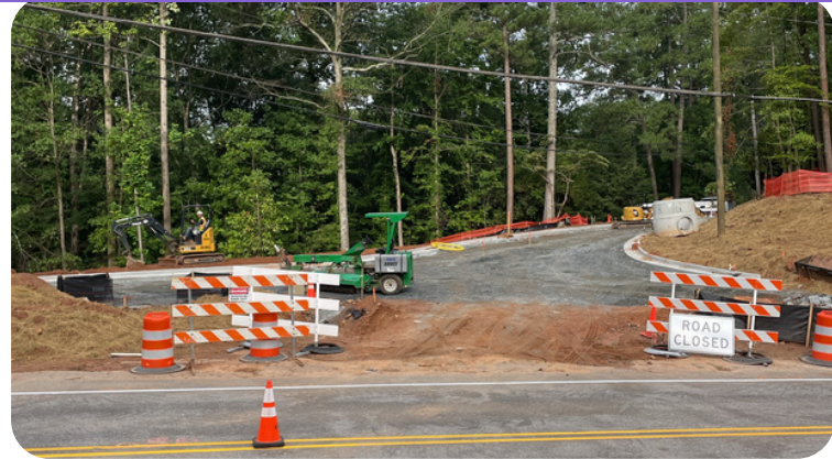
⚡ TS106 Old Powers Ferry Road - Riverview Intersection Site Work
