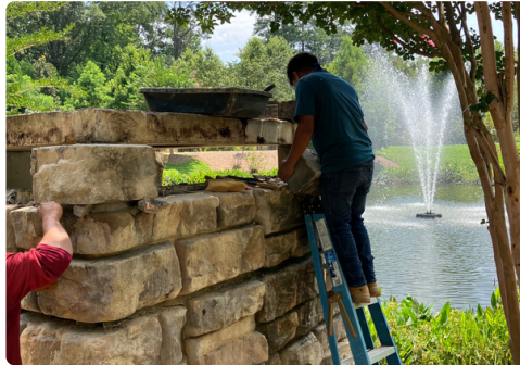
Marsh Creek Before and after stone repair
