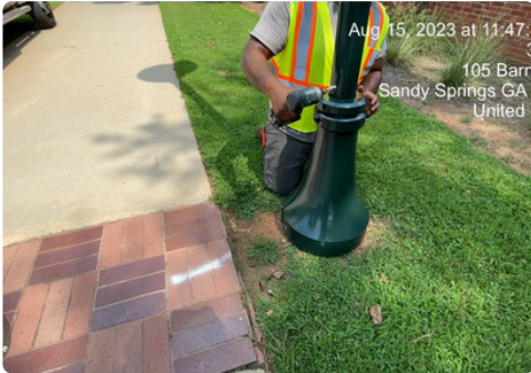
Johnson Ferry Road Finishing touches on the pedestrian lighting project
