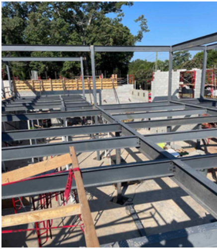
Photo Description (left to right): Structural Steel Second Floor, Continuing Installation of Exterior CMU, Interior CMU Installation at the First Floor Decon Area
