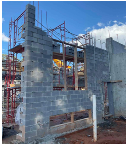
Photo Description (left to right): Structural Steel Second Floor, Continuing Installation of Exterior CMU, Interior CMU Installation at the First Floor Decon Area
