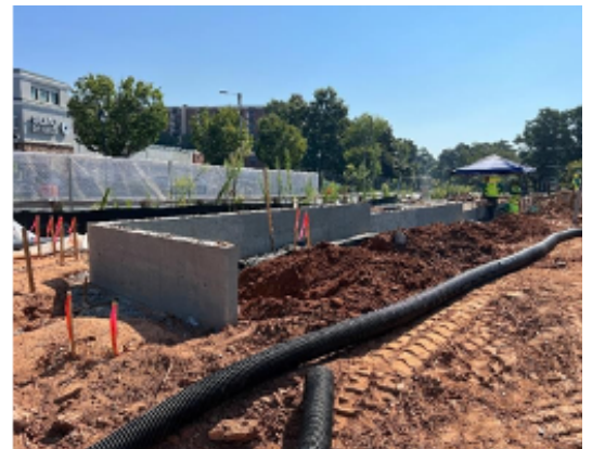
Photo Description (left to right): Restarted work at original Jack-n-Bore pit, Completed pour of Johnson Ferry lower wall, installed toe drain
