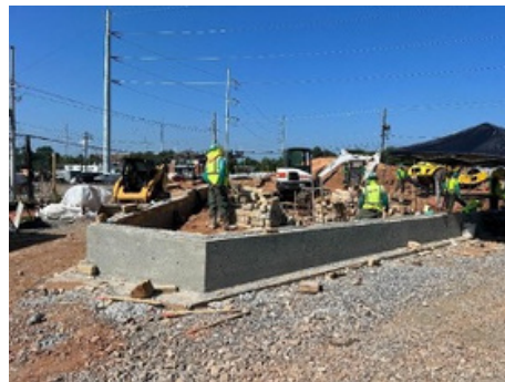
Photo Description (left to right): Completed veneer on 45 deg wall, finishing veneer along Mt. Vernon Wall, beginning veneer along Johnson Ferry lower wall
