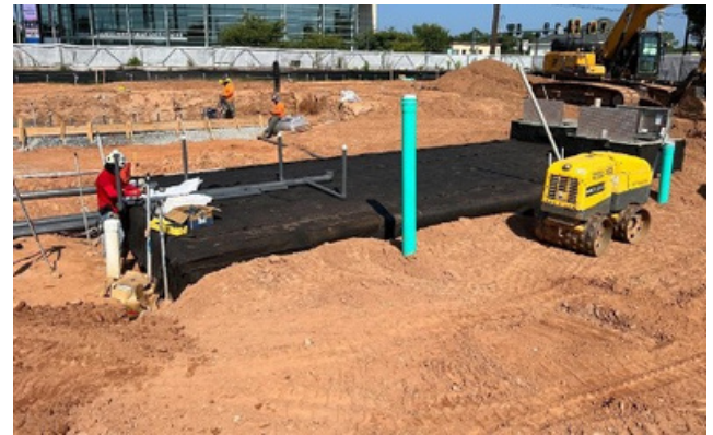
Photo Description (left to right): Prepping first fountain slab with plumbing roughed, Backfill of vault, Waterproof lid, install vault hatches
