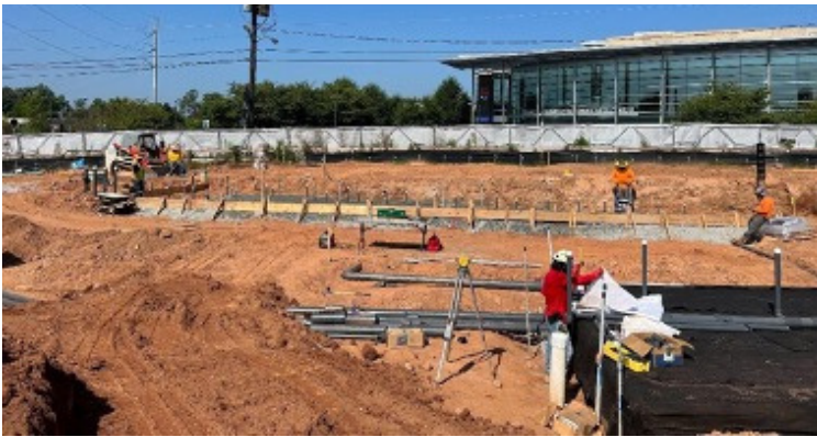
Photo Description (left to right): Prepping first fountain slab with plumbing roughed, Backfill of vault, Waterproof lid, install vault hatches
