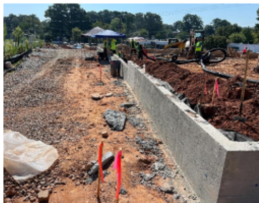
Photo Description (left to right): Restarted work at original Jack-n-Bore pit, Completed pour of Johnson Ferry lower wall, installed toe drain
