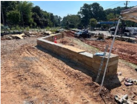
Photo Description (left to right): Completed veneer on 45 deg wall, finishing veneer along Mt. Vernon Wall, beginning veneer along Johnson Ferry lower wall
