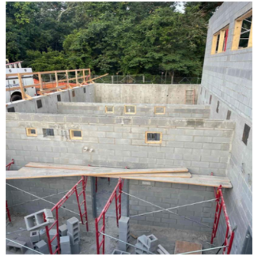
Photo Description (left to right): Structural Steel Second Floor, Continuing Installation of Exterior CMU, Interior CMU Installation at the First Floor Decon Area
