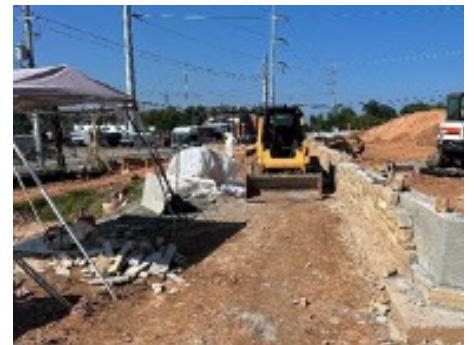
Photo Description (left to right): Completed veneer on 45 deg wall, finishing veneer along Mt. Vernon Wall, beginning veneer along Johnson Ferry lower wall
