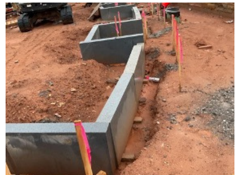
Photo Description (left to right): Rain delay seen from accumulation in utility pit, Continued veneer along Johnson Ferry lower wall, Began granite curb install
