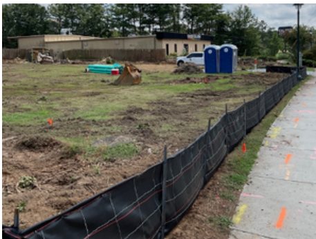
Photo Description (left to right): Silt Fence Installed Around the Perimeter of the Site, Continued Clearing and Grubbing
