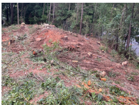
Photo Description (left to right): Continued Clearing and Grubbing, Continued To Clear Trees
