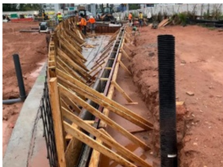
Photo Description (left to right): Forming fountain walls, Completed first flagpole installation
