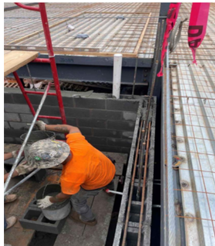
Photo Description (left to right): Elevated Slab on Deck Prep at the Second Floor, Continuing Installation of Interior CMU, Continuing in-wall Rough-in and CMU
