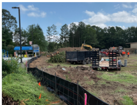
Photo Description (left to right): Silt Fence Installed Around the Perimeter of the Site, Continued Clearing and Grubbing
