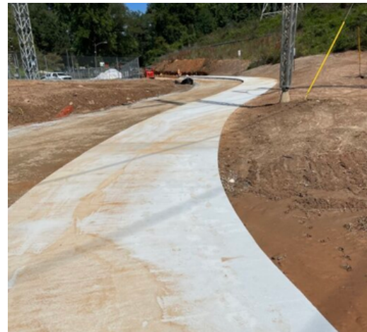
Springway Trail - Concrete from the drive to the wall.
