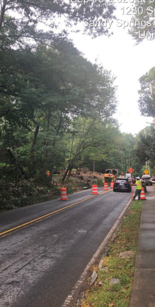
TS111 Spalding Drive at Pitts Road clearing underway.
