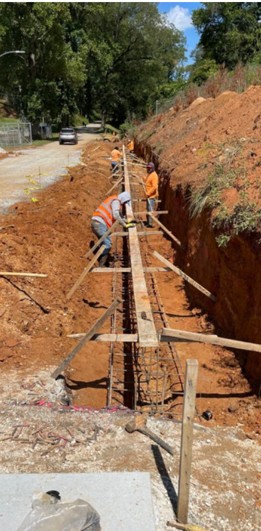
Springway Trail - installation of concrete wall.
