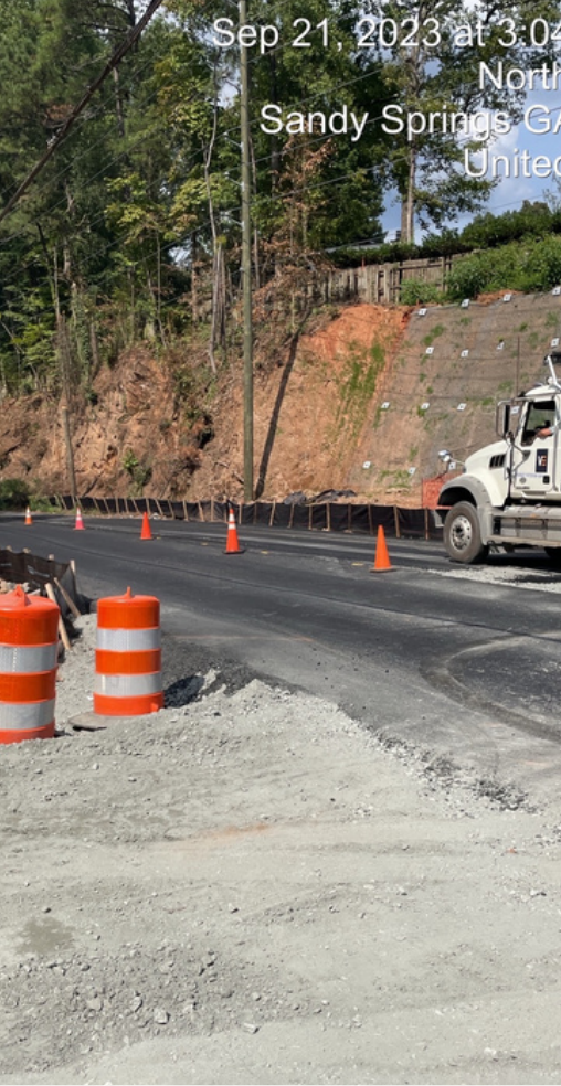
PW TS106 Northside Old Powers Ferry Riverview Intersection site work
