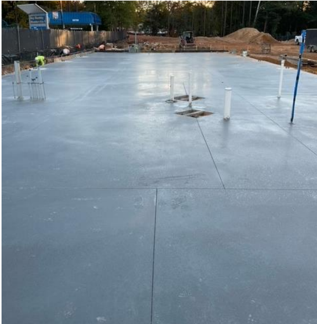
Completed Pouring The SOG
