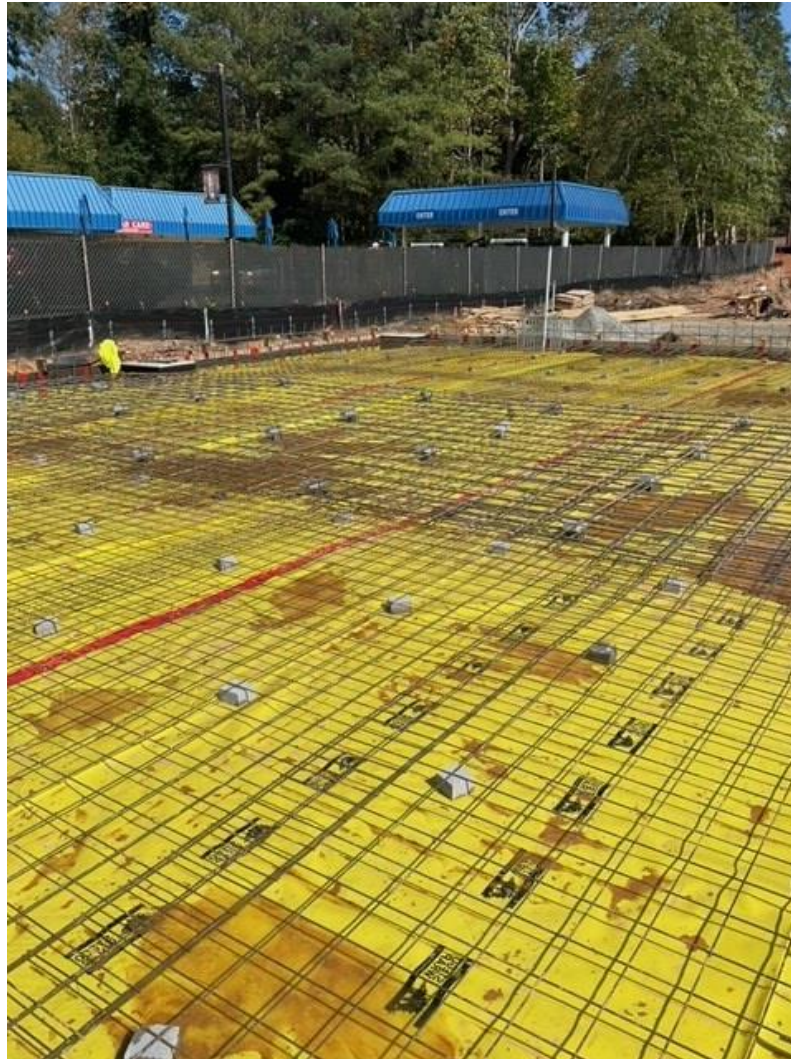
Prep For Slab
