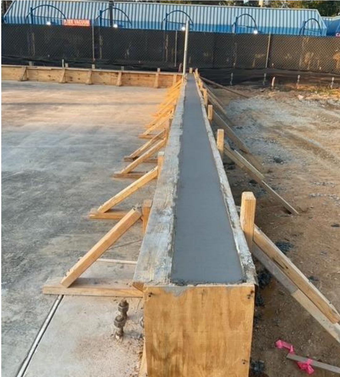
Formed And Poured The Stem Wall
