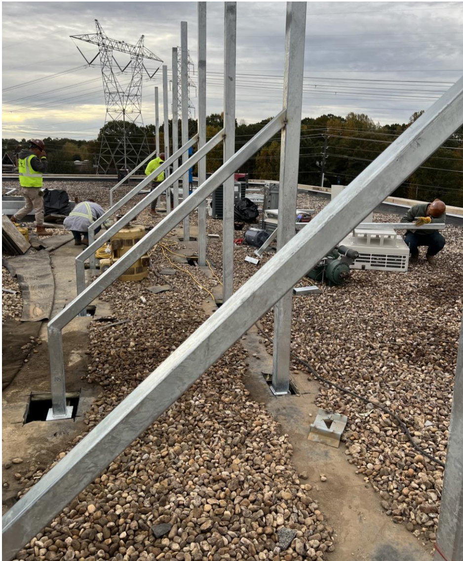
Begin Roof Steel For The Screen Wall
