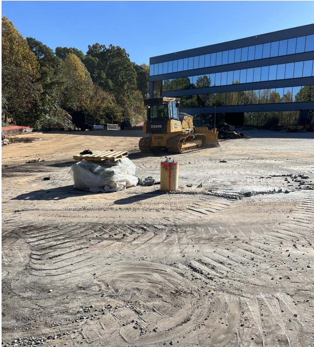
Begin Asphalt Demo
