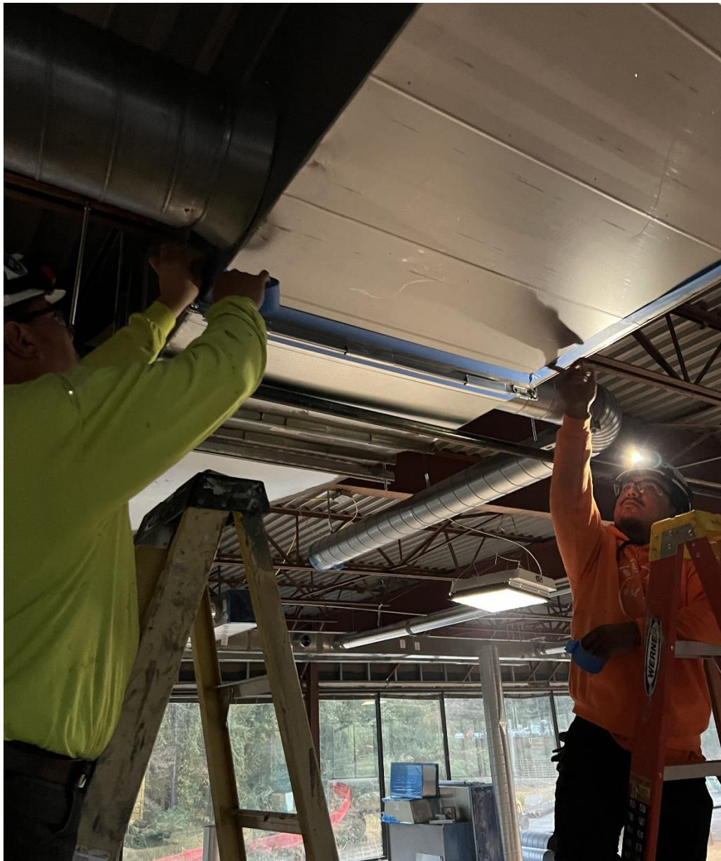
Continue Joist Augmentation on Level 2
