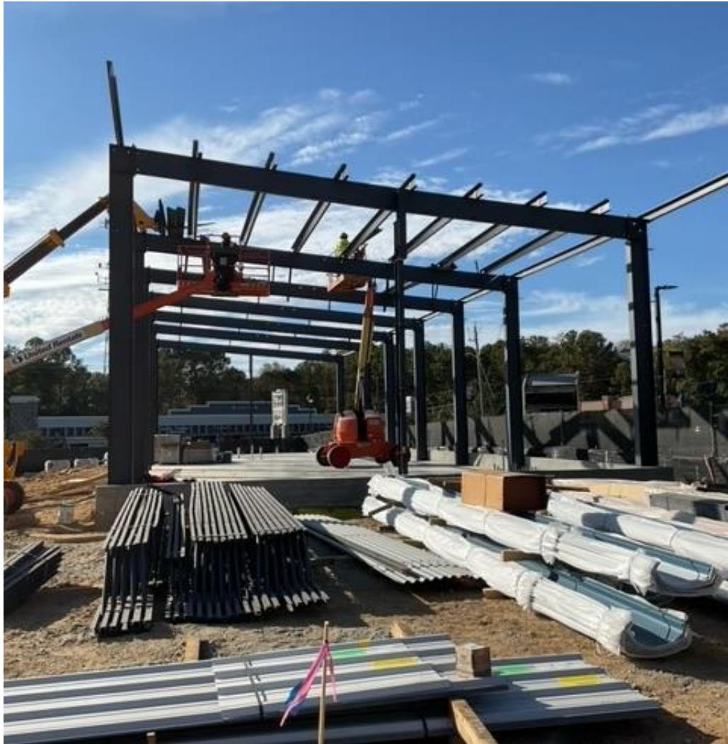
Completed Main Frame
