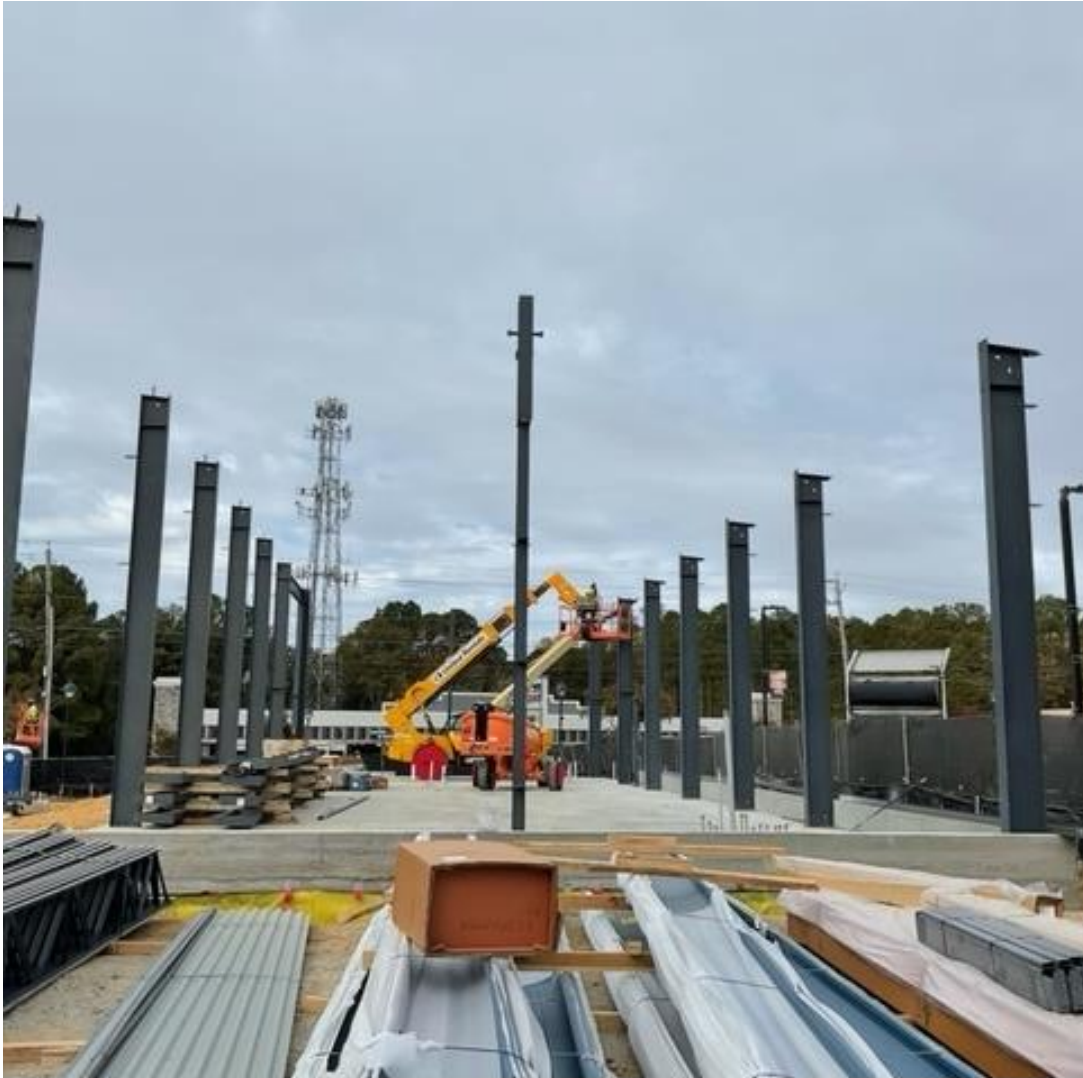
Began Erecting The Steel Columns
