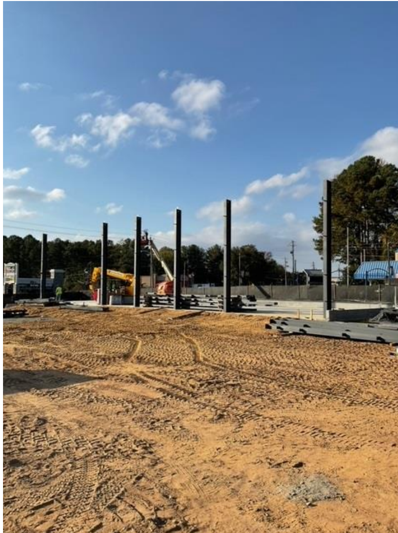
Began Erecting The Steel Columns
