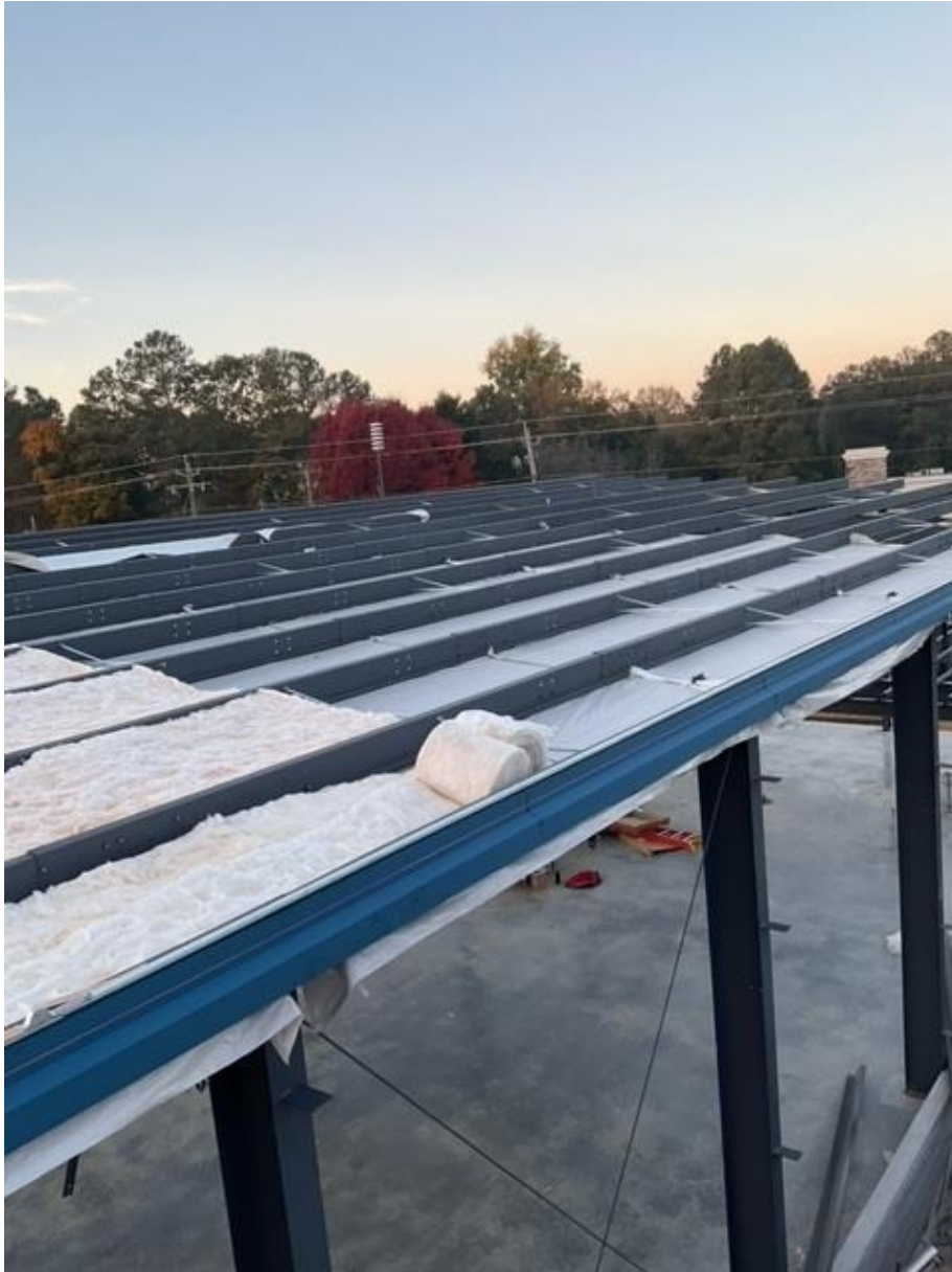
Began Installing The Insulation
