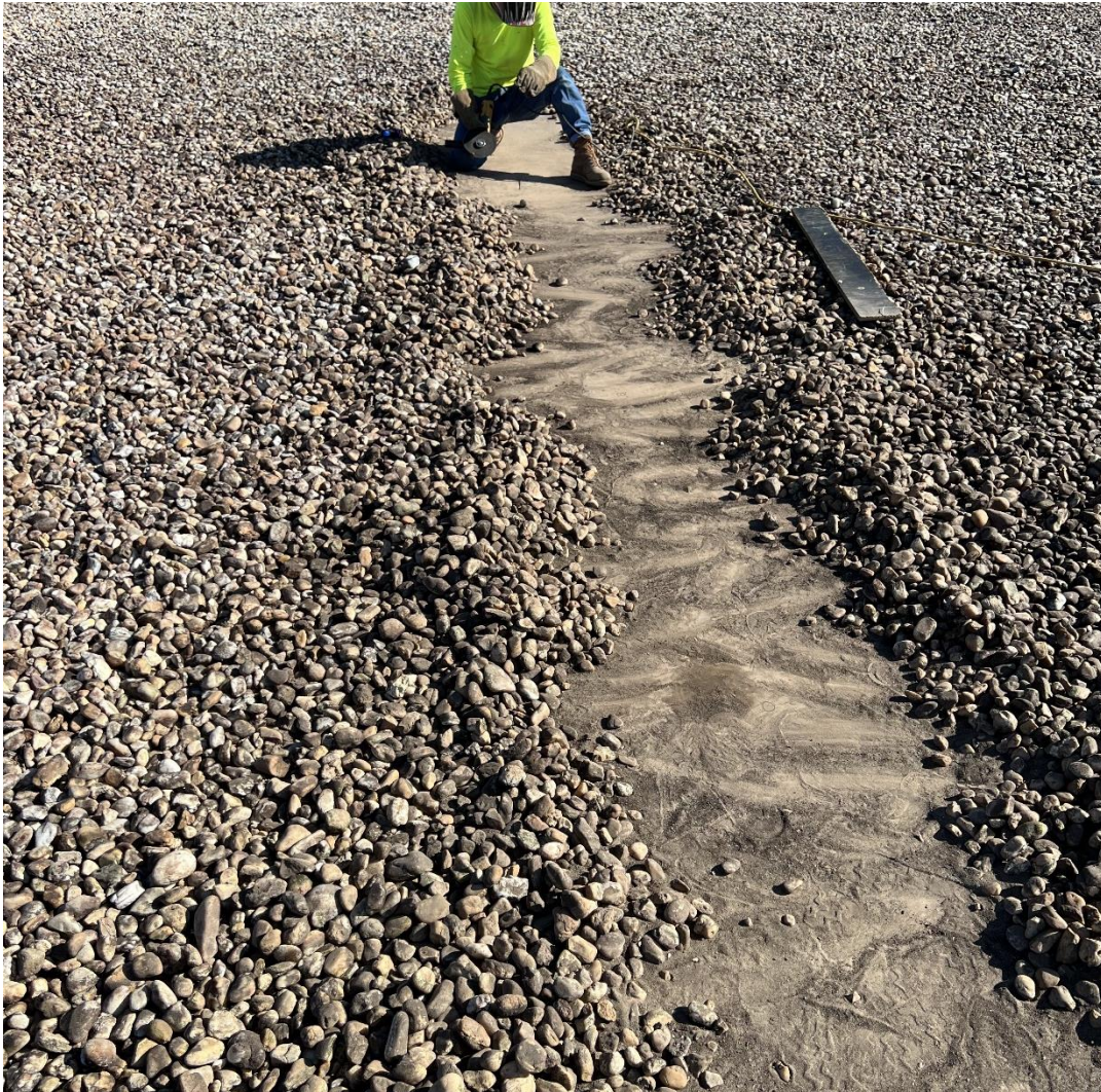
Clearing stone for Roof Steel For Screen Wall
