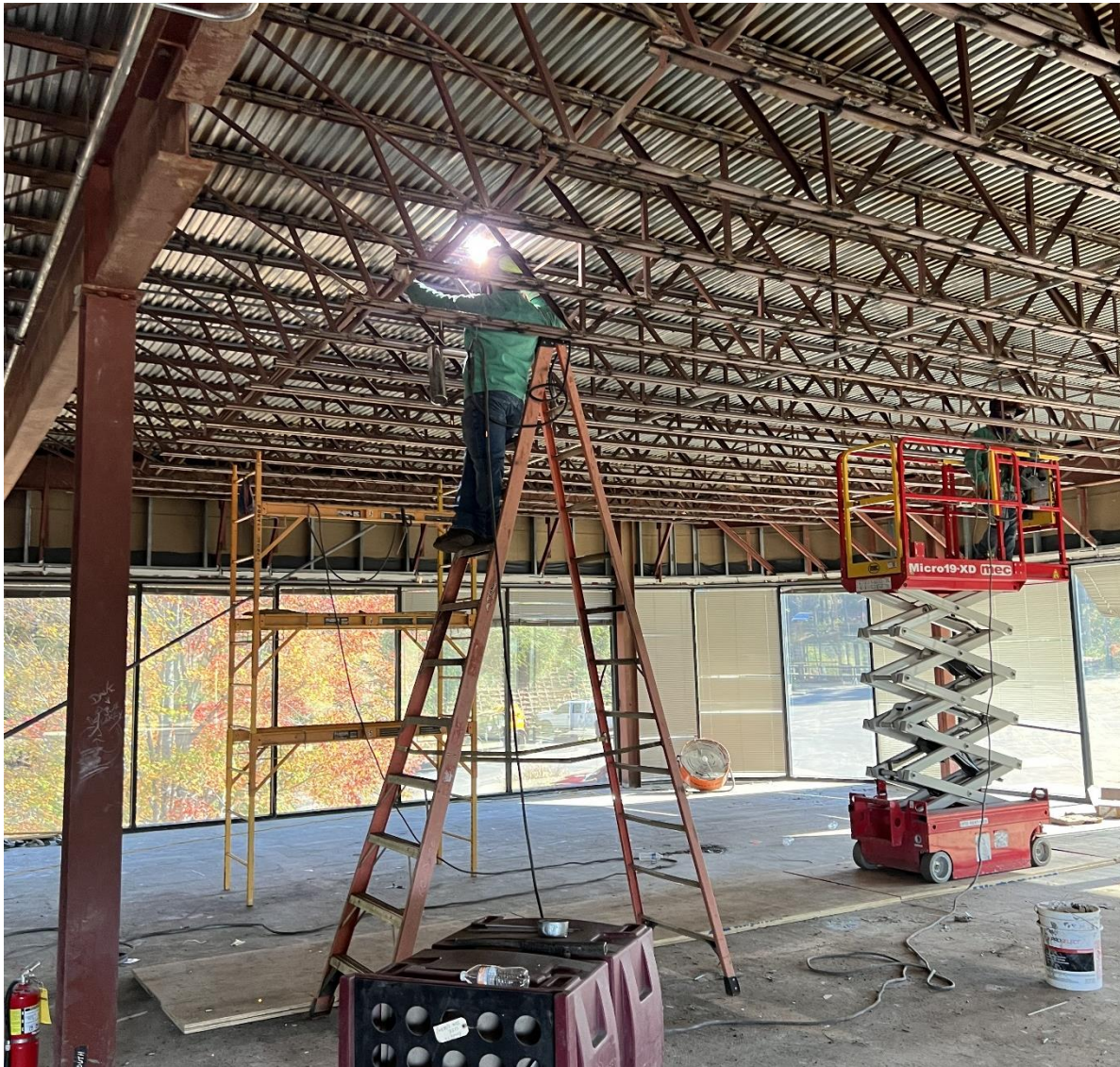
Joist Augmentation on Level 2
