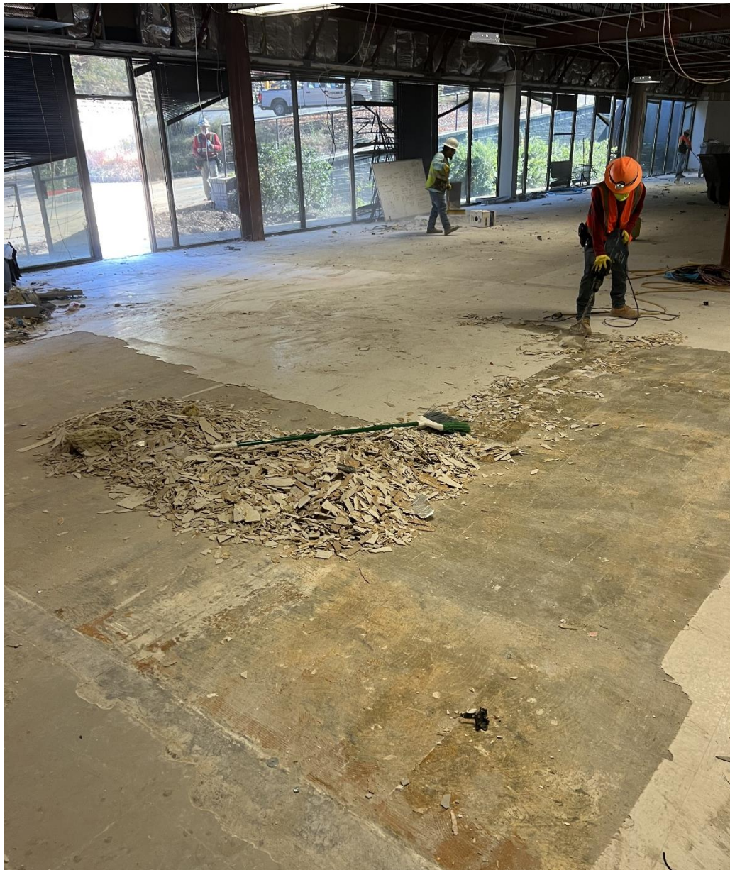
Final Demolition Clean And Completion
