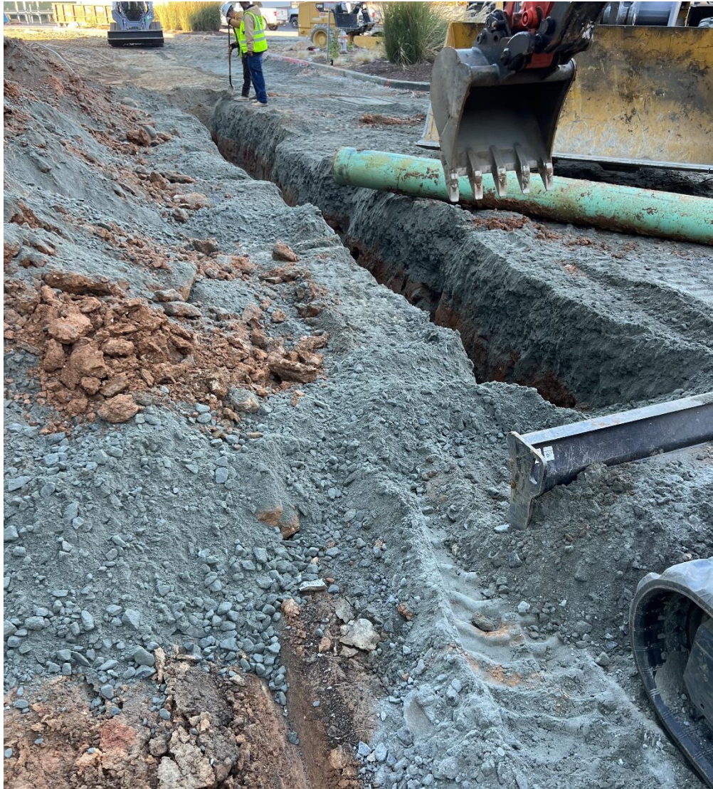
Begin Demolition Of Existing Utilities
