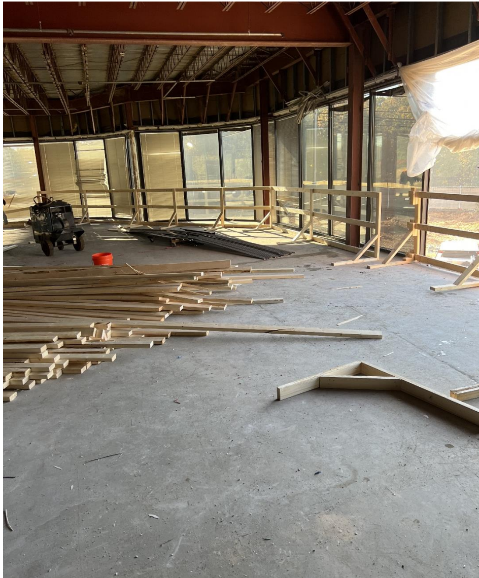
Install Safety Rails Along The Interior
