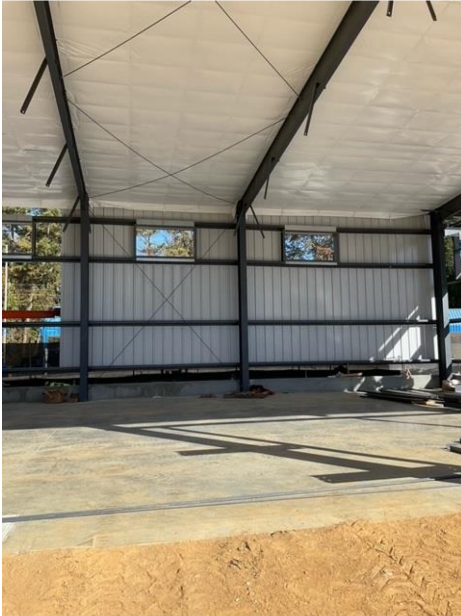
Installation of Wall Paneling
