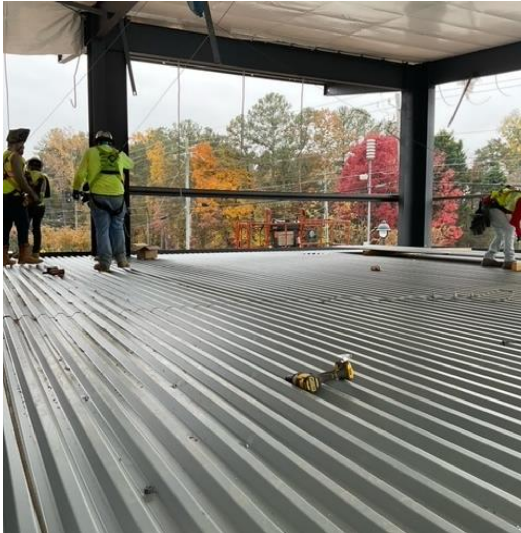
Begin Wall Framing And Paneling
