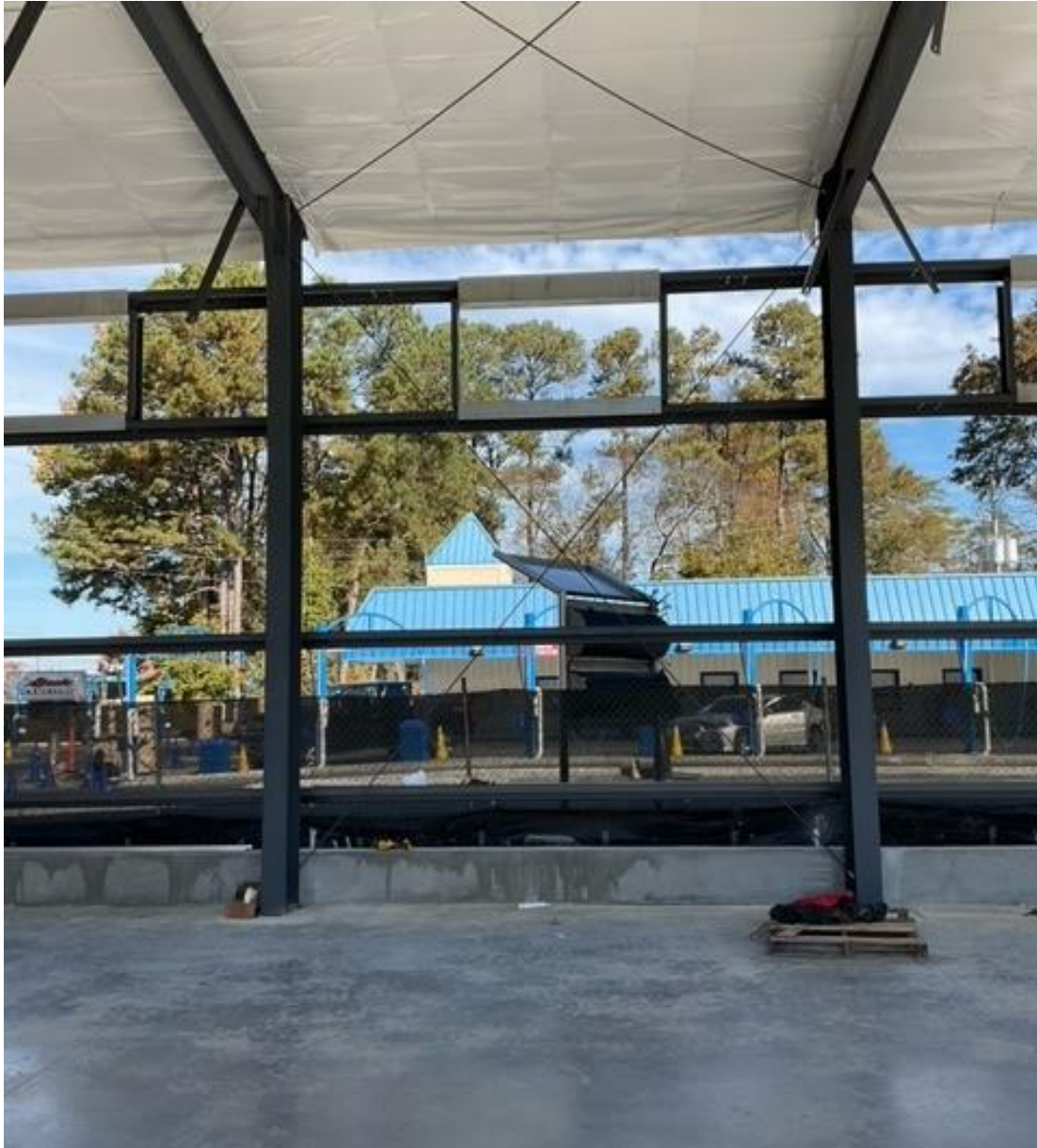
Began Framing Out Openings
