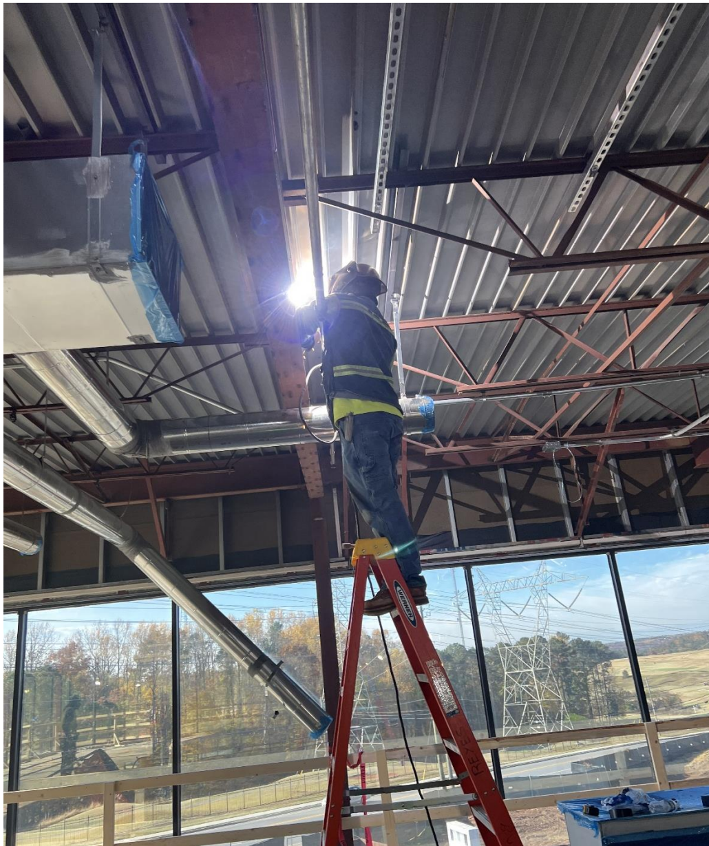
Joist Augmentation Re-Work
