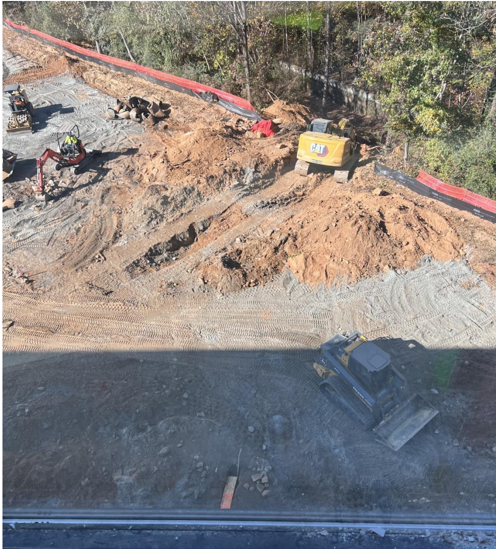
Exterior Site Demolition
