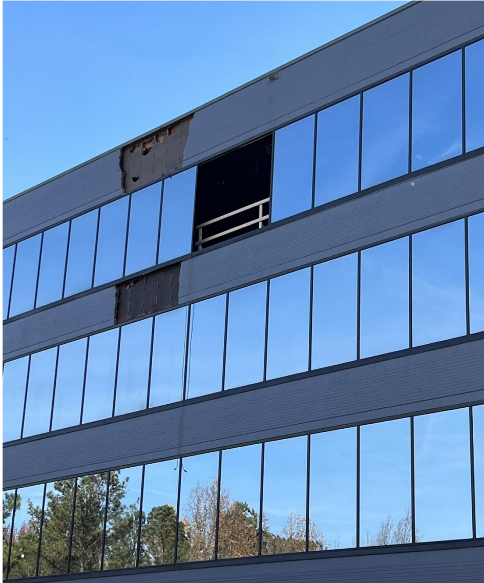
Begin Exterior Demolition At SW End Of The Building
