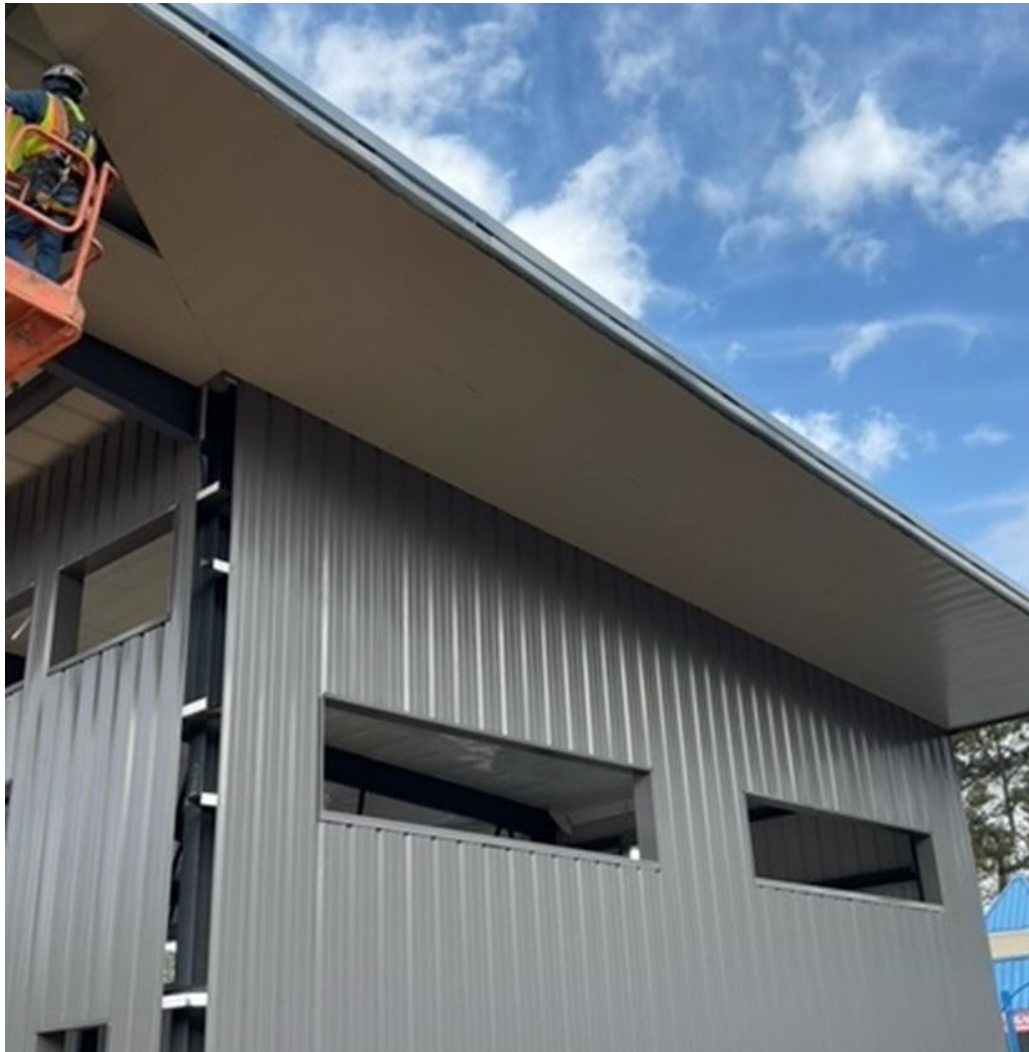
Finished Soffit Installation
