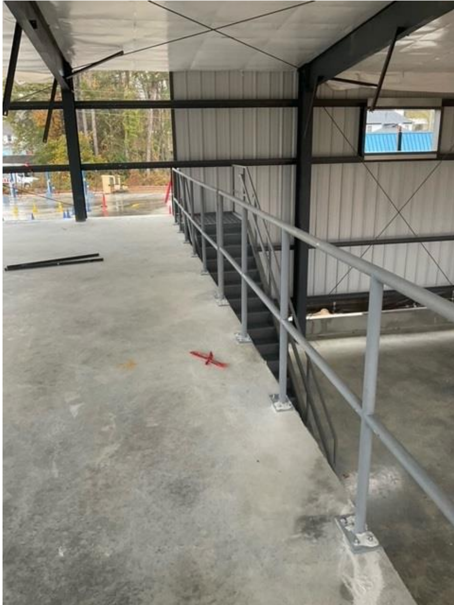
Completed Setting the Stairs & Railings @ Mezzanine
