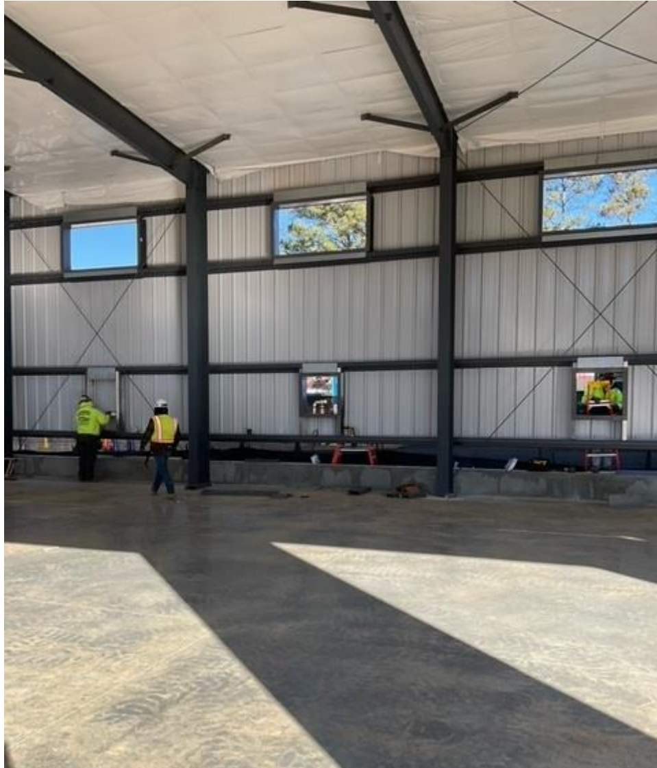
Continue Trim Work inside PEMB
