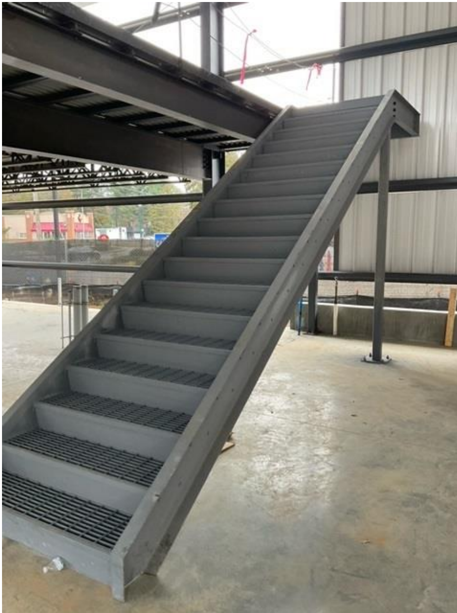
Began Setting The Stairs
