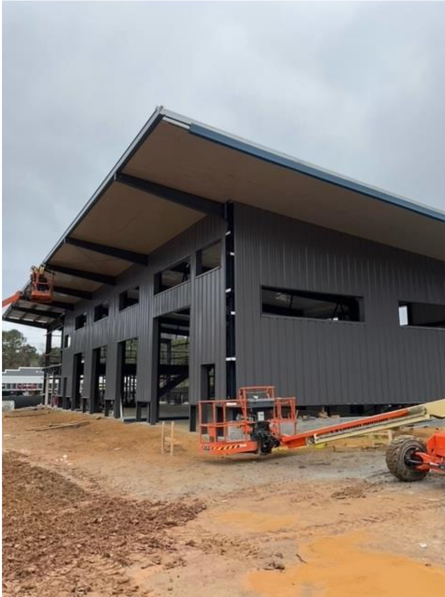
Completed Framing Out The Rough Openings On The West Side
