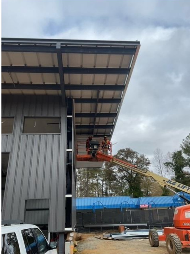
Began Installing Soffit on PEMB
