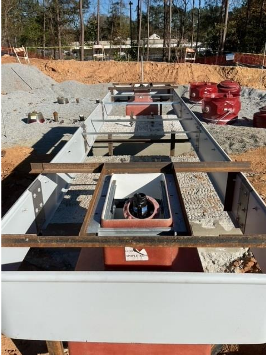
Prepping for Fuel Island
