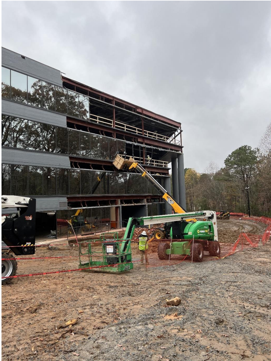
Continue Exterior Demo of Brick/Glass/Lintel/Kicker - North Face
