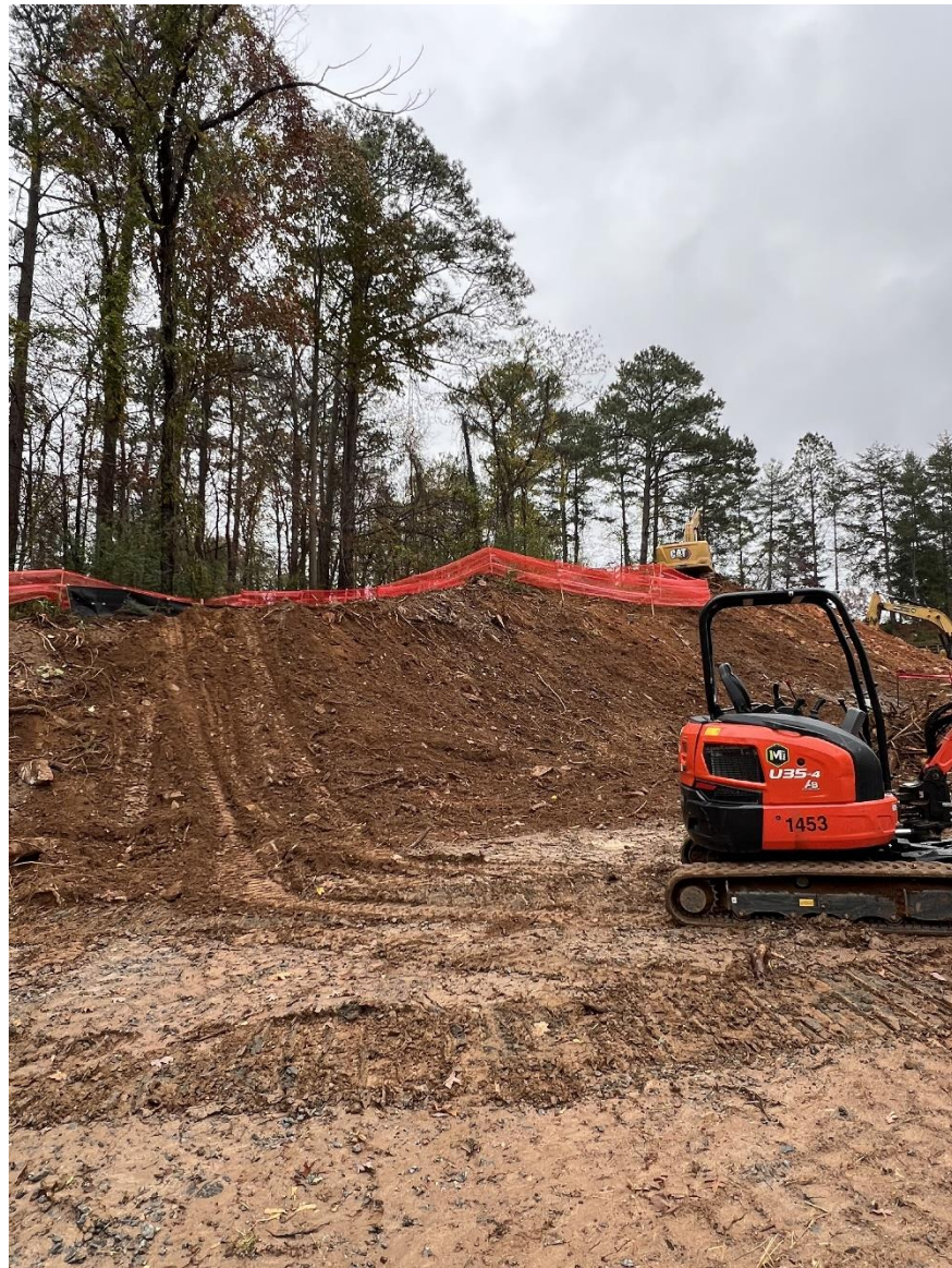
Begin Demo & Grading at Retaining Wall
