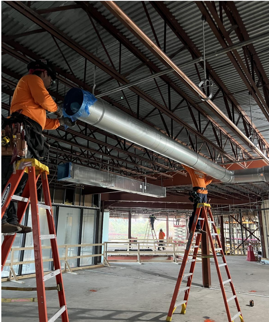
Continue Mecanical PIU/VAV Rough-In
