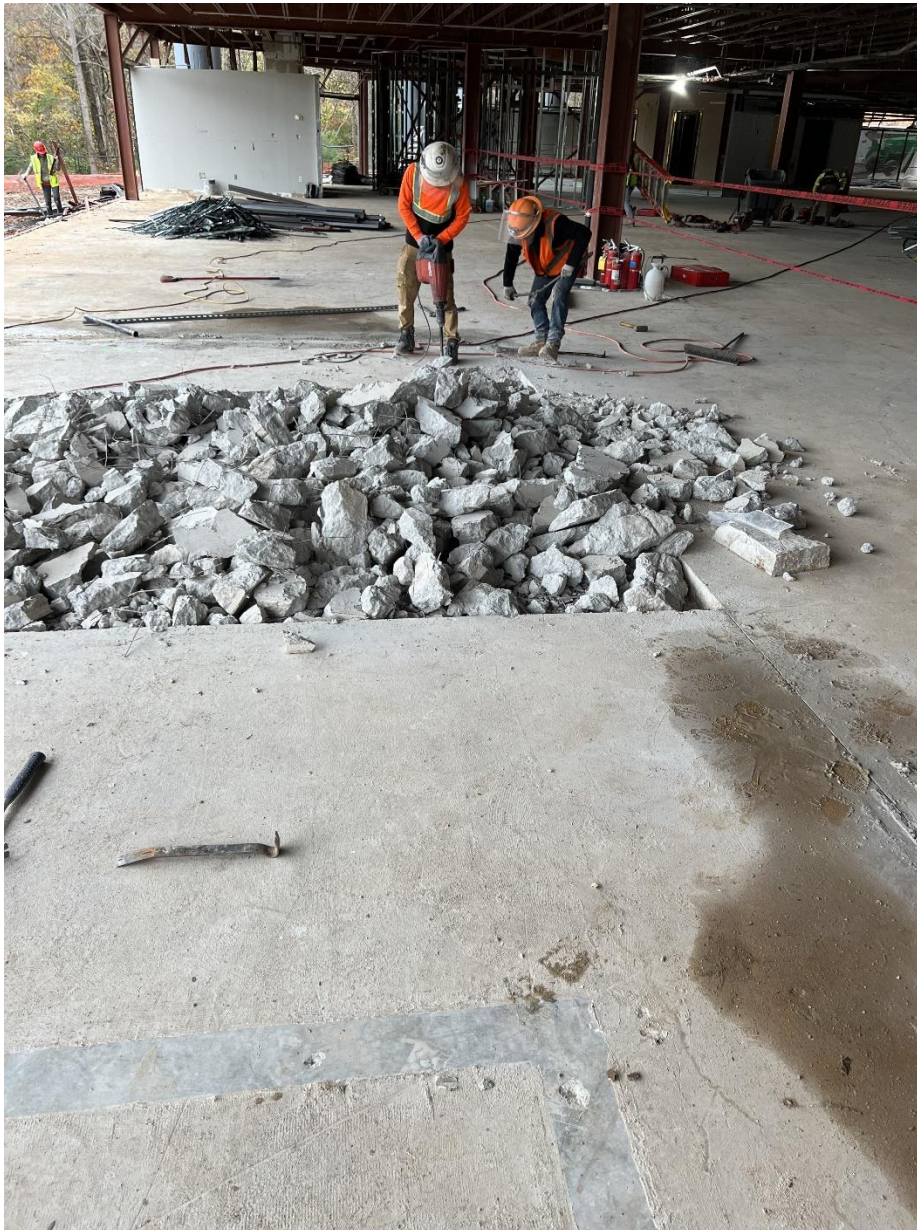
Continue Demolition Of The Basement Slab
