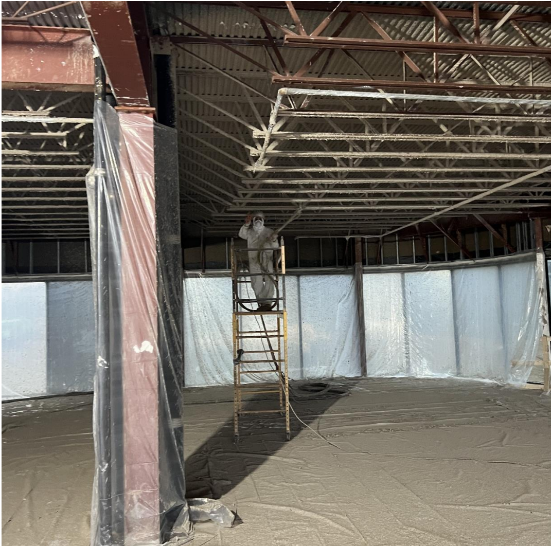
Continue Fireproofing On Level 1
