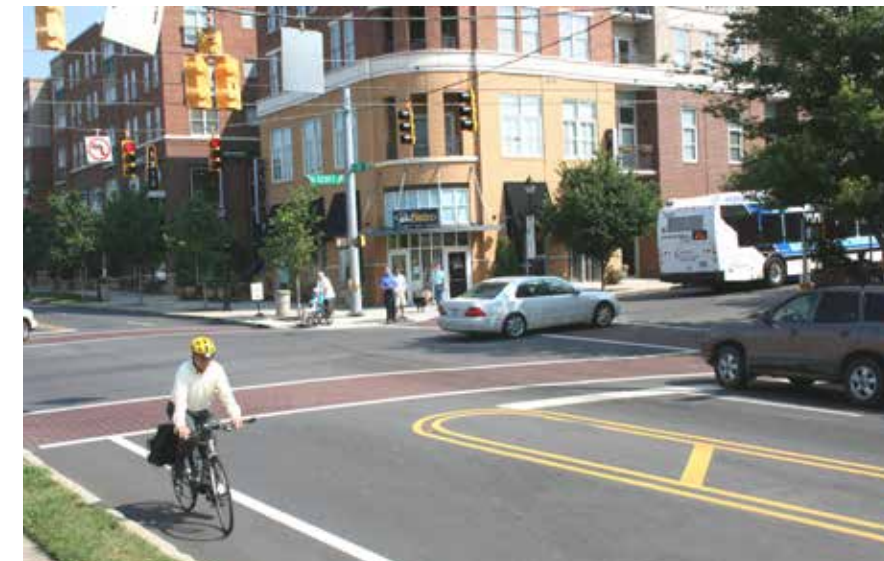
Redevelopment incorporating a connected street grid and multimodal transportation options. (Source: Complete Streets via Flickr)
