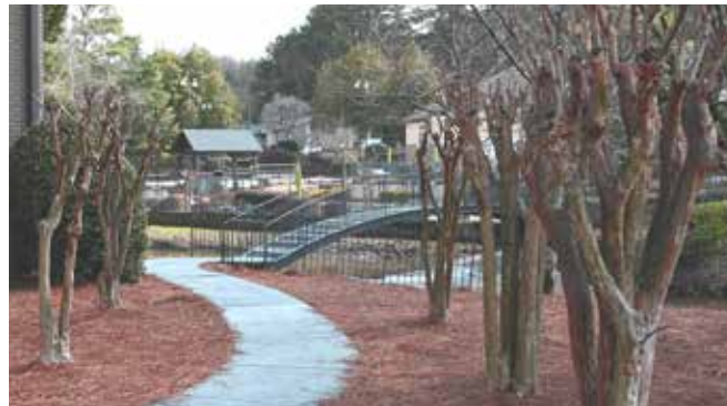
Trail and pedestrian bridge crossing Long Island Creek
