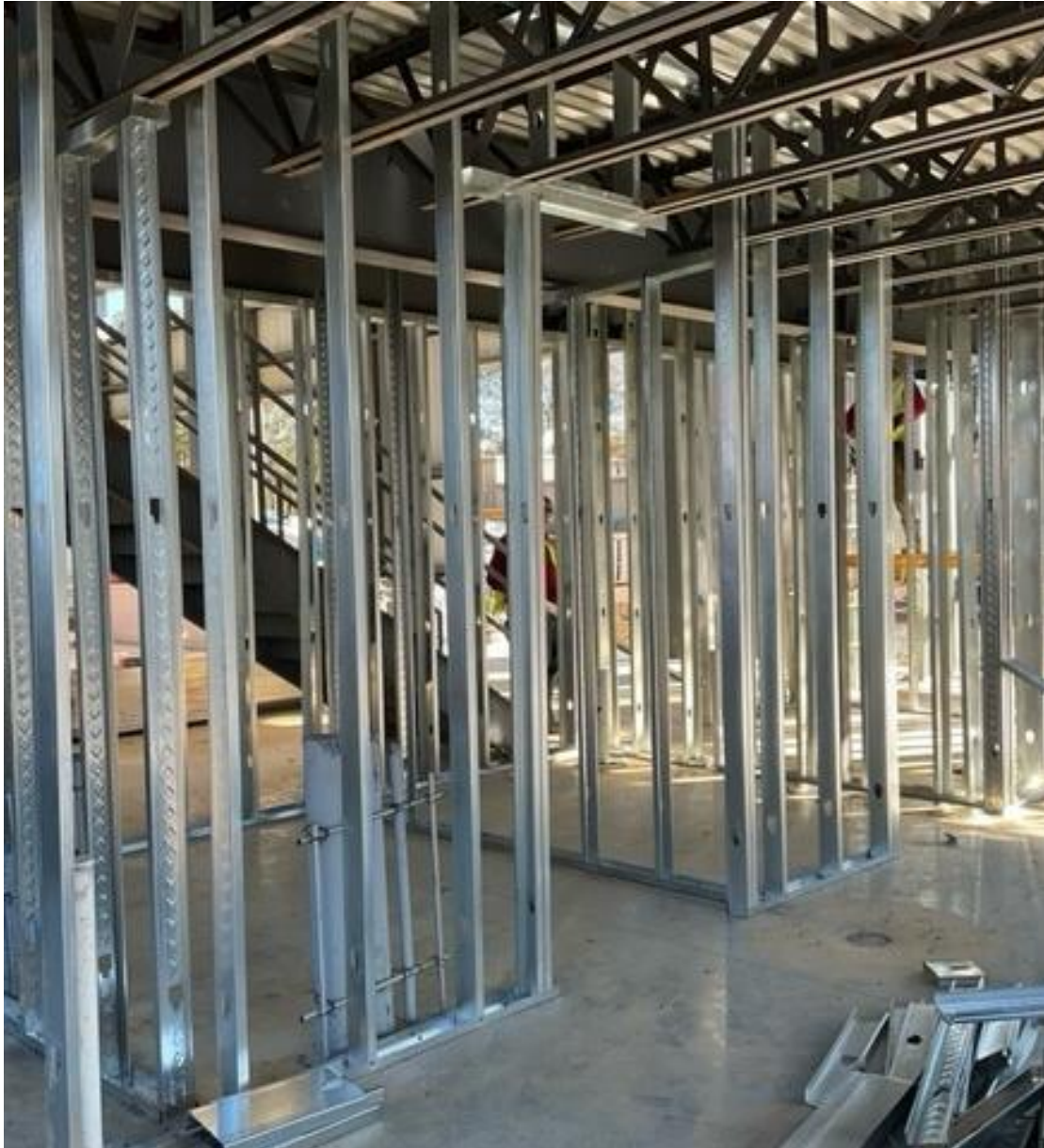
Continuing Interior Framing
