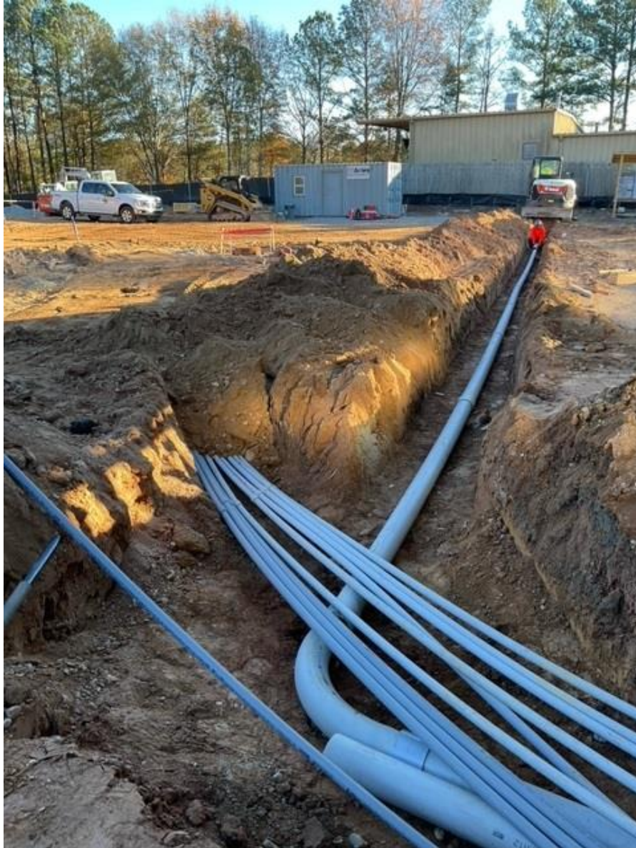
Begin Running The Electrical Conduit Through The Site
