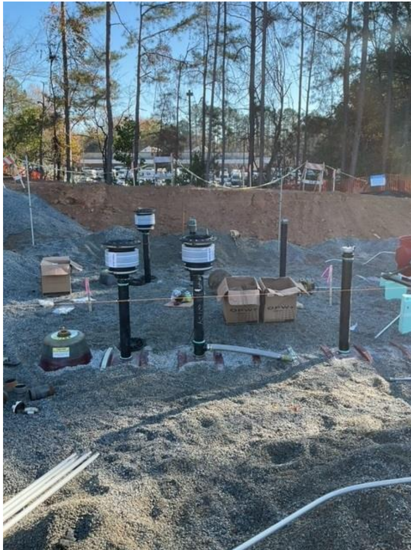
Begin Installing Fuel Station Vent System
