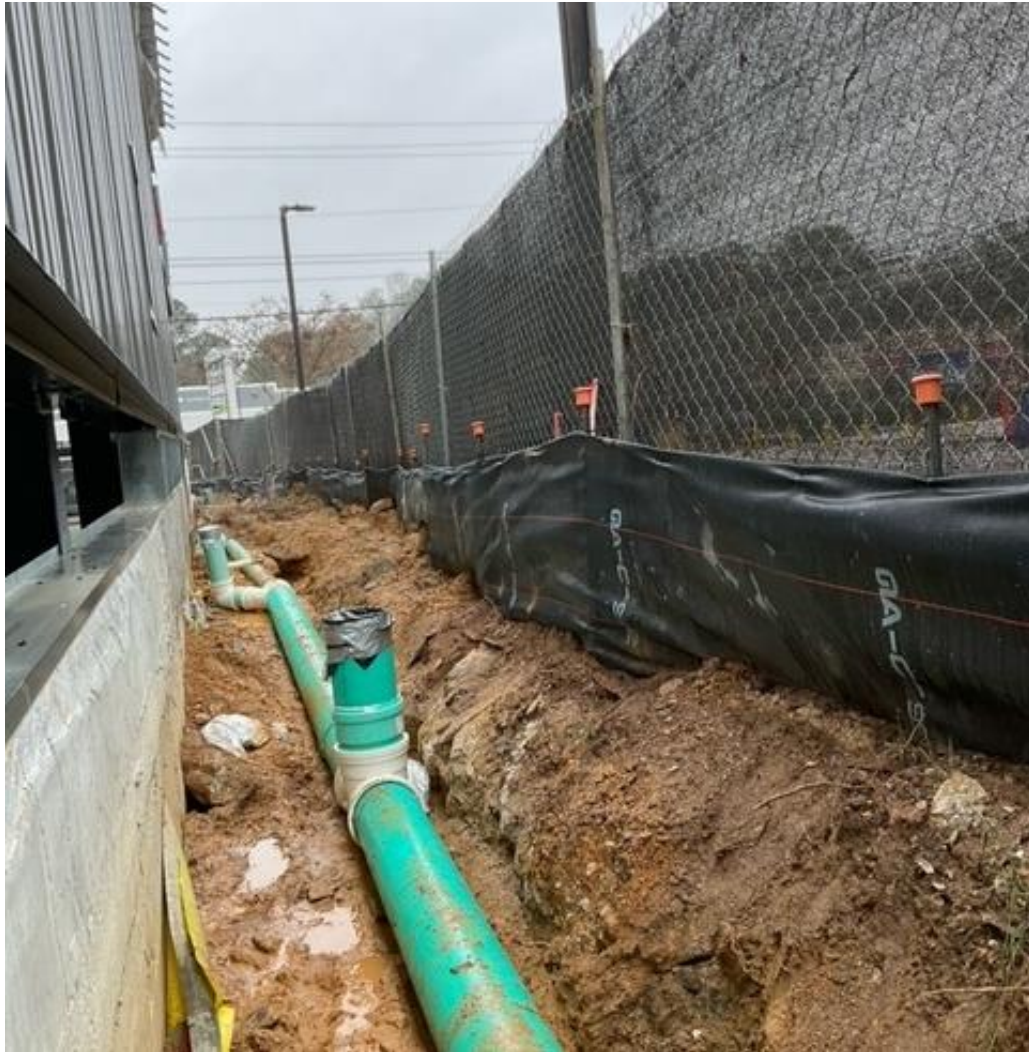
Installed Storm Drain
