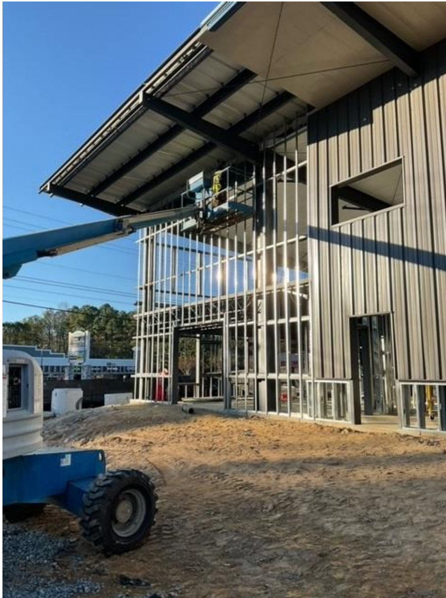
Began Exterior Sheathing
