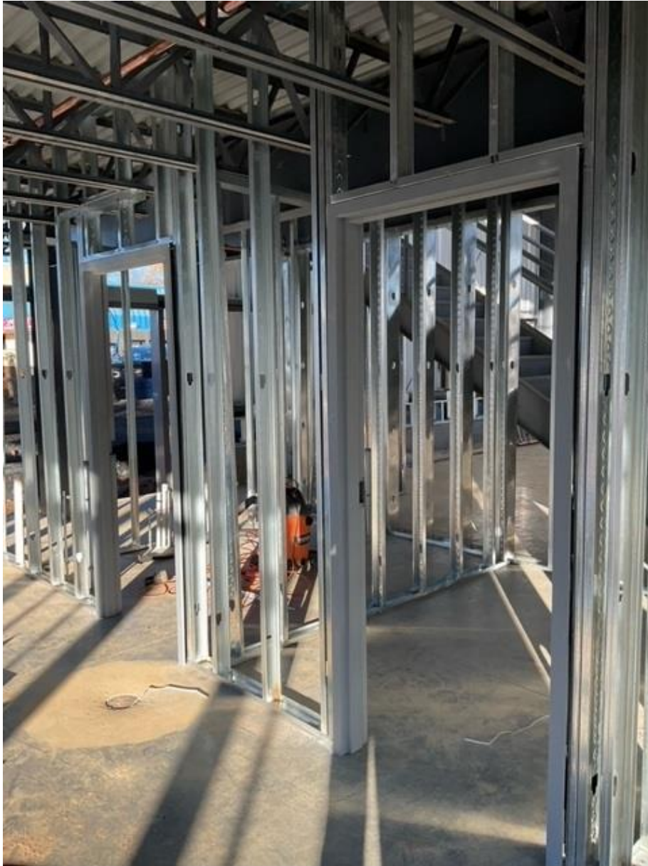
Door Frames Installed
