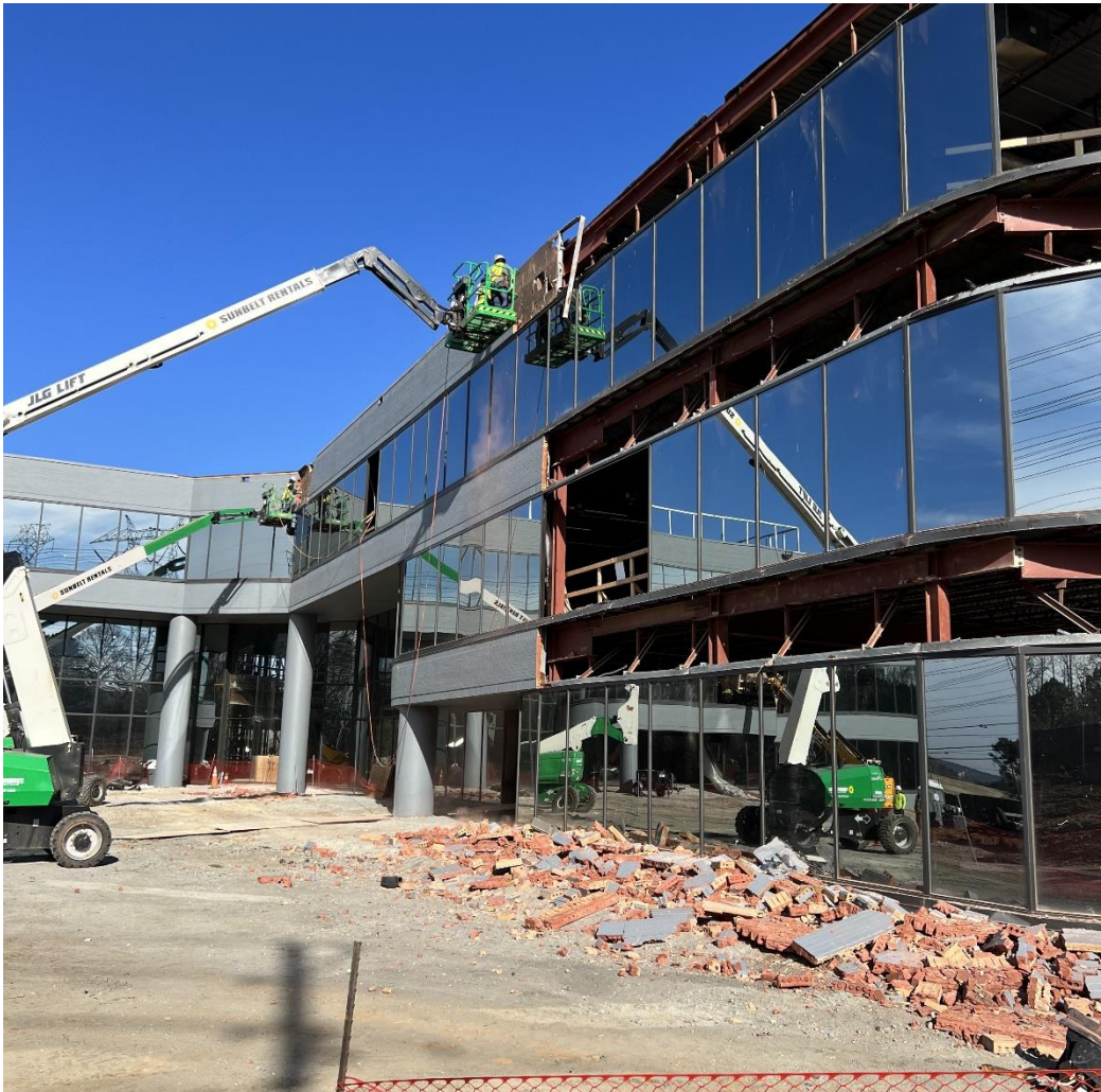
Continue Exterior Demo Of Brick/Glass/Lintel/Kicker
