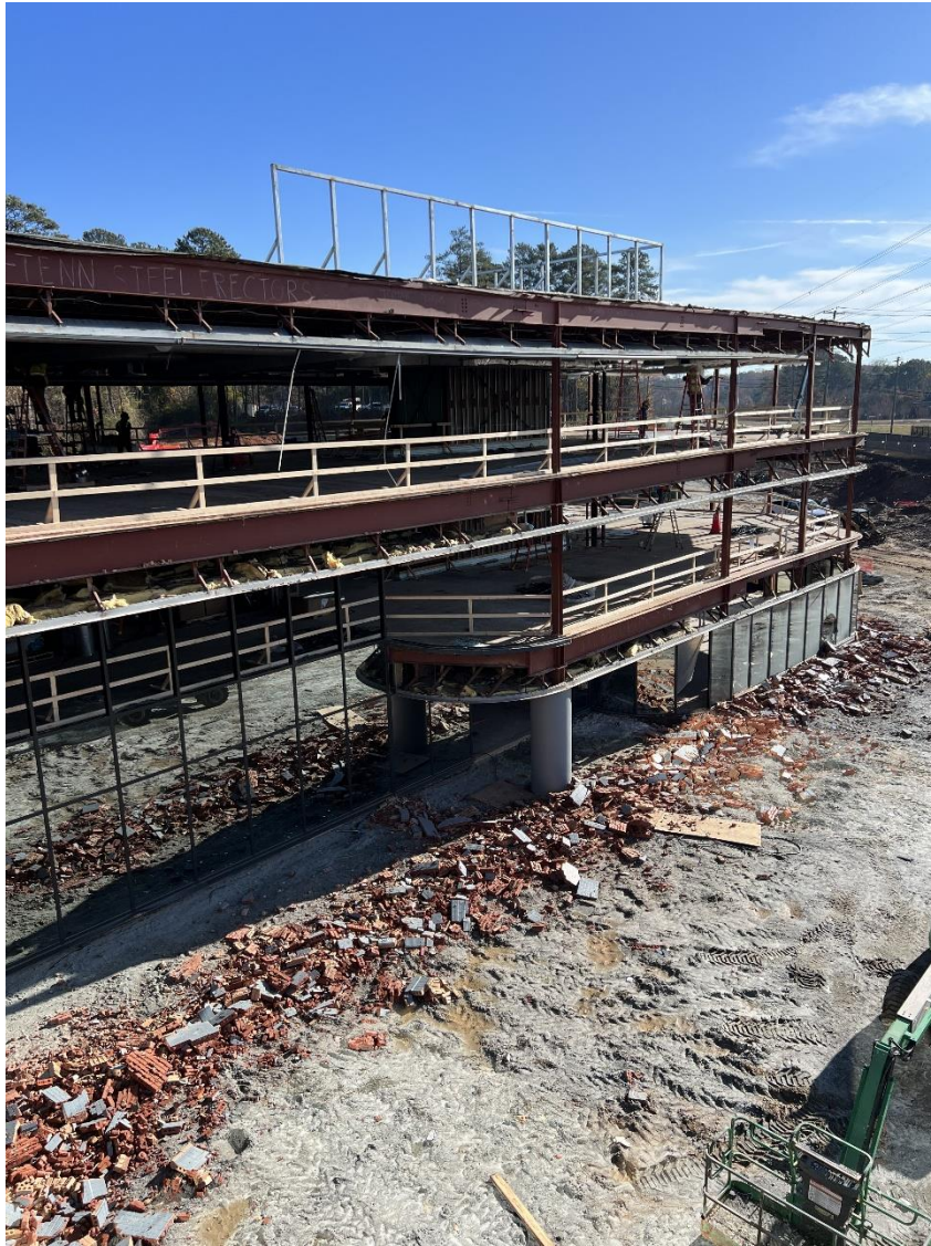
Continue Exterior Demo of Brick/Glass/Lintel/Kicker
