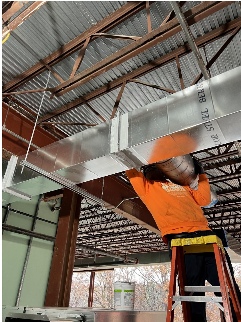
Mechanical Overhead Rough-in On Level 2
