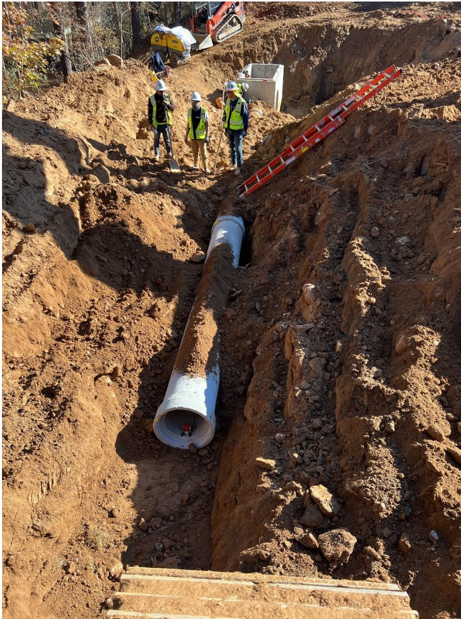
Continue Installing U/G Utilities
