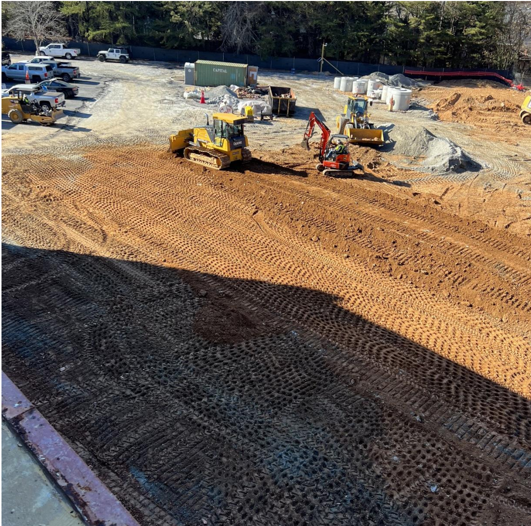
Continue Grading At Sally Port
