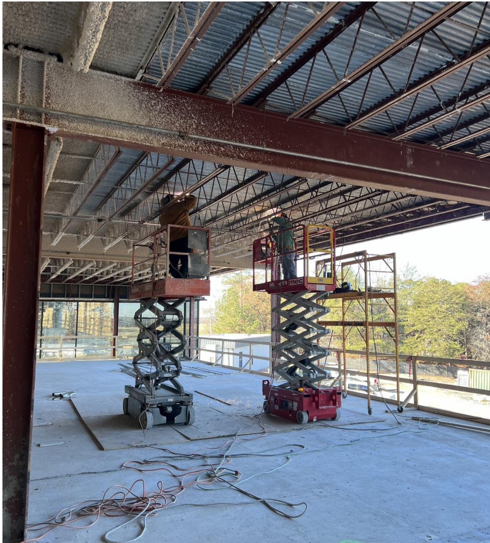
Joist Augmentation On Level 1
