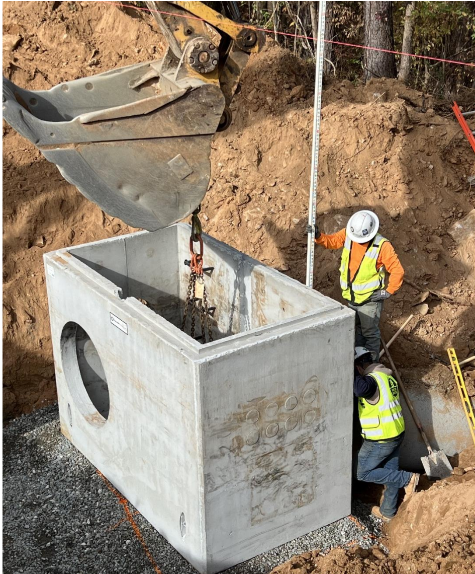
Continue Installing U/G Utilities
