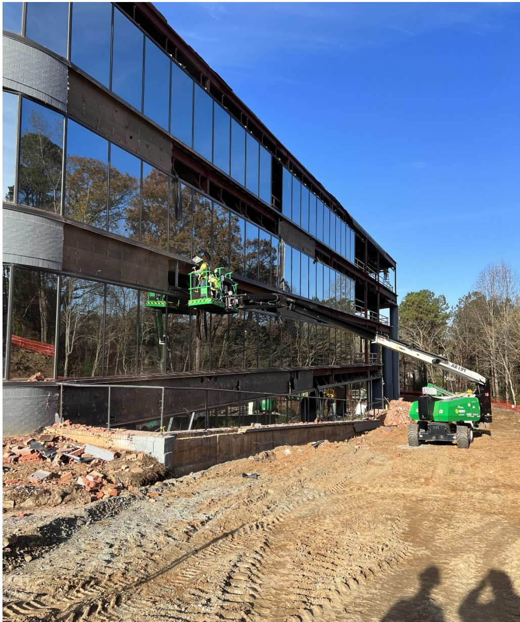
Continue Exterior Demo Brick/Glass/Lintel/Kicker - North Face
