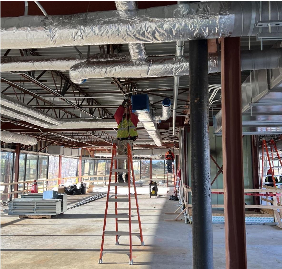
Continue Mechanical PIU/VAV Rough-In On Level 3
