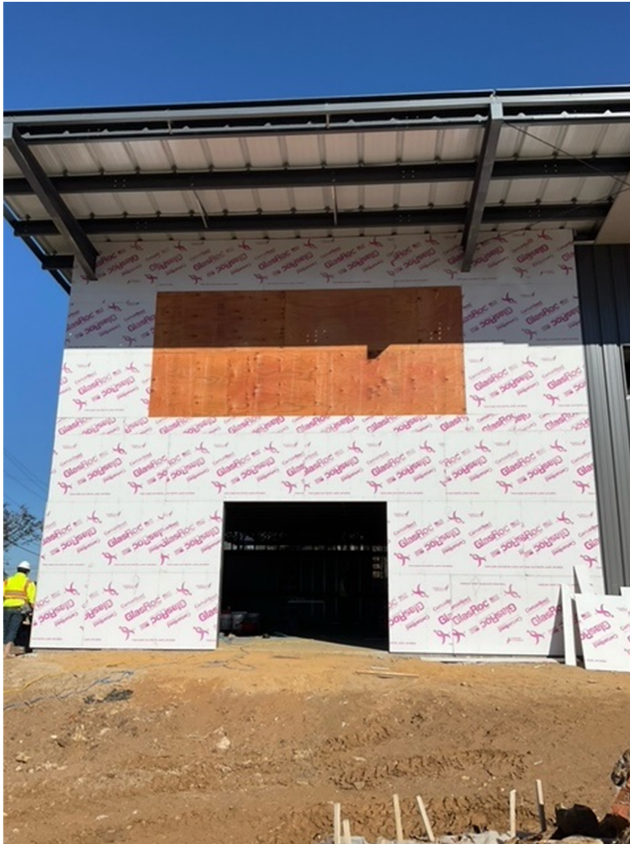
Completed Exterior Sheathing
