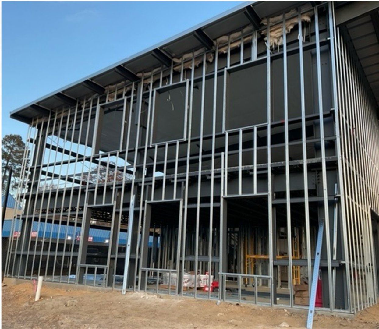
Exterior Framing Installed
