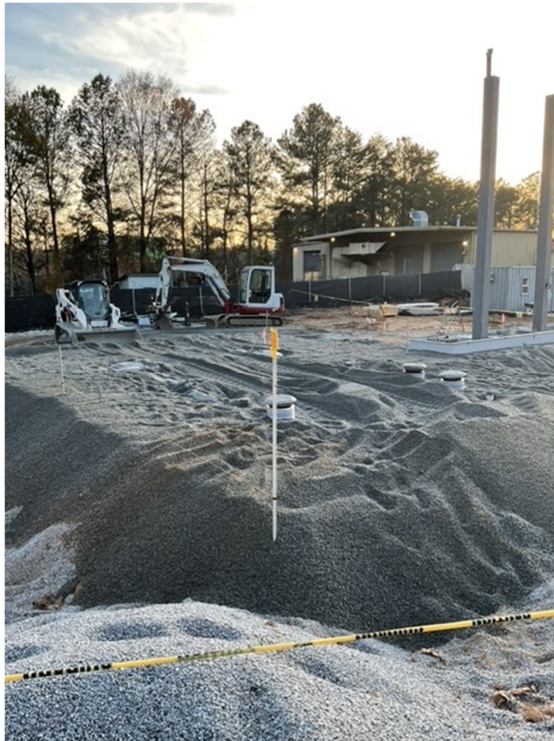
Tank Pad And Fuel Island Canopy Backfilled With Stone
