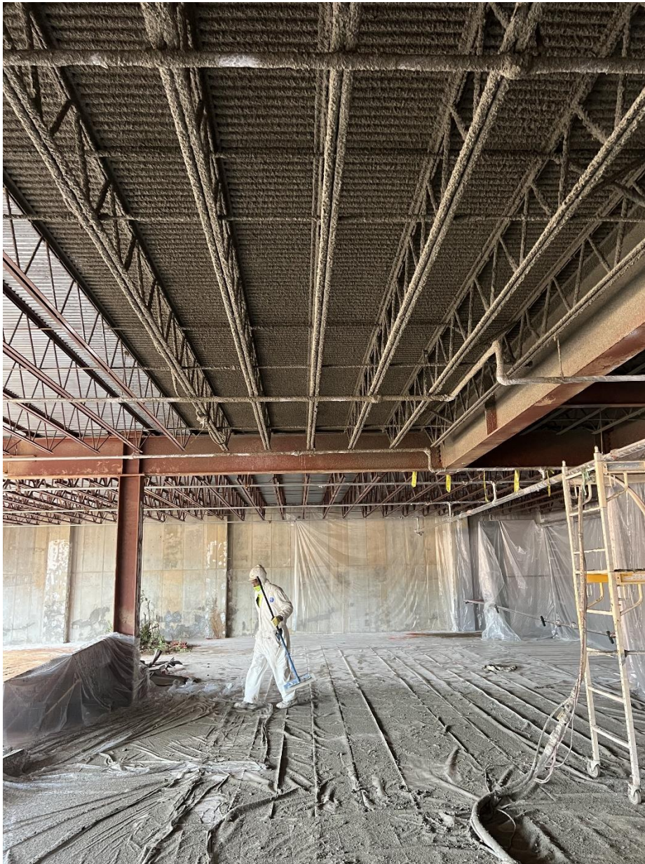
Begin Fireproofing Basement
