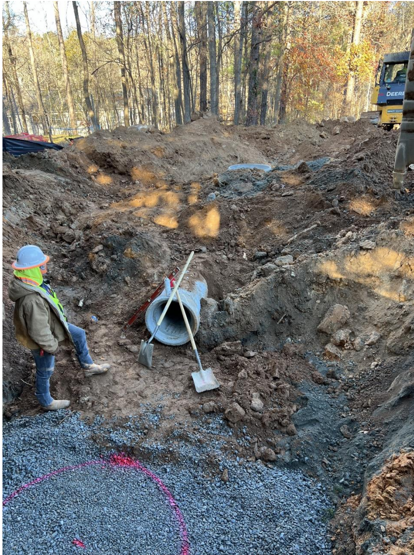
Continue Installing U/G Utilities
