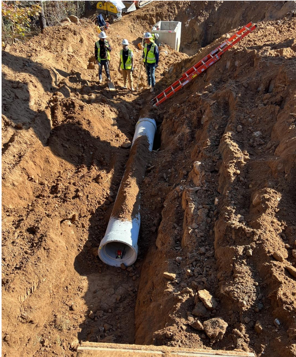
Continue Installing U/G Utilities
