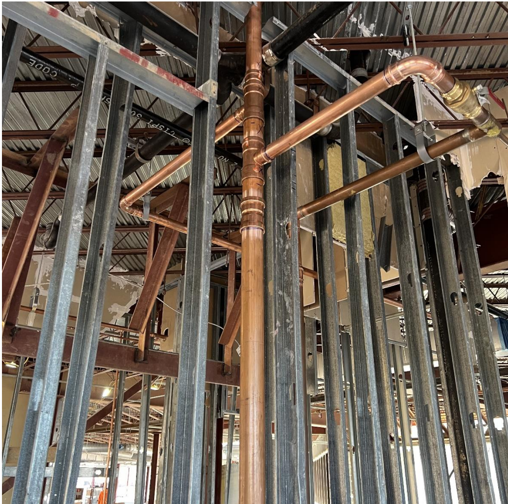
Continue Plumbing Overhead Rough-In On Level 3
