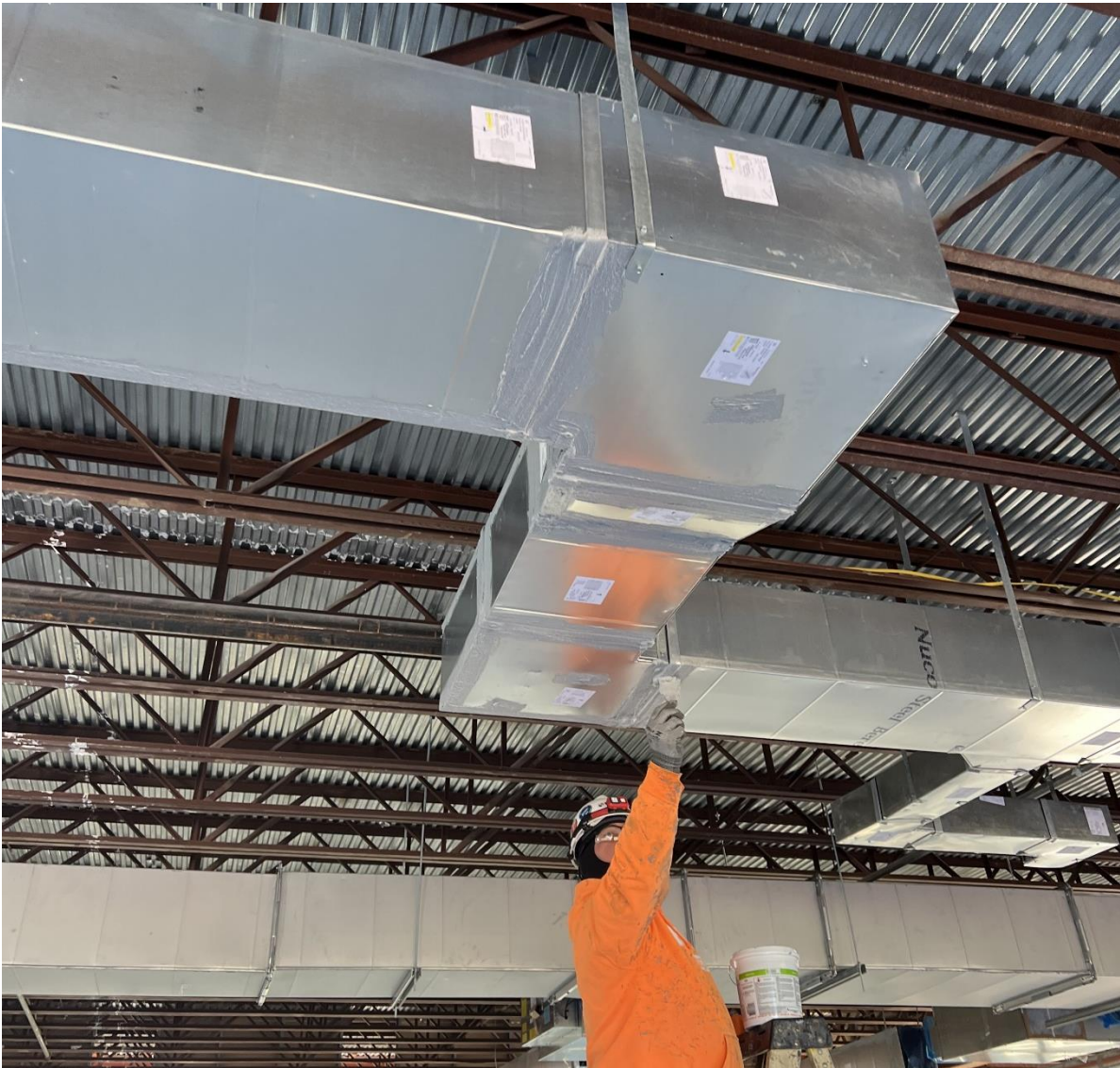
Continue Mechanical PIU/VAV Rough-In On Level 3
