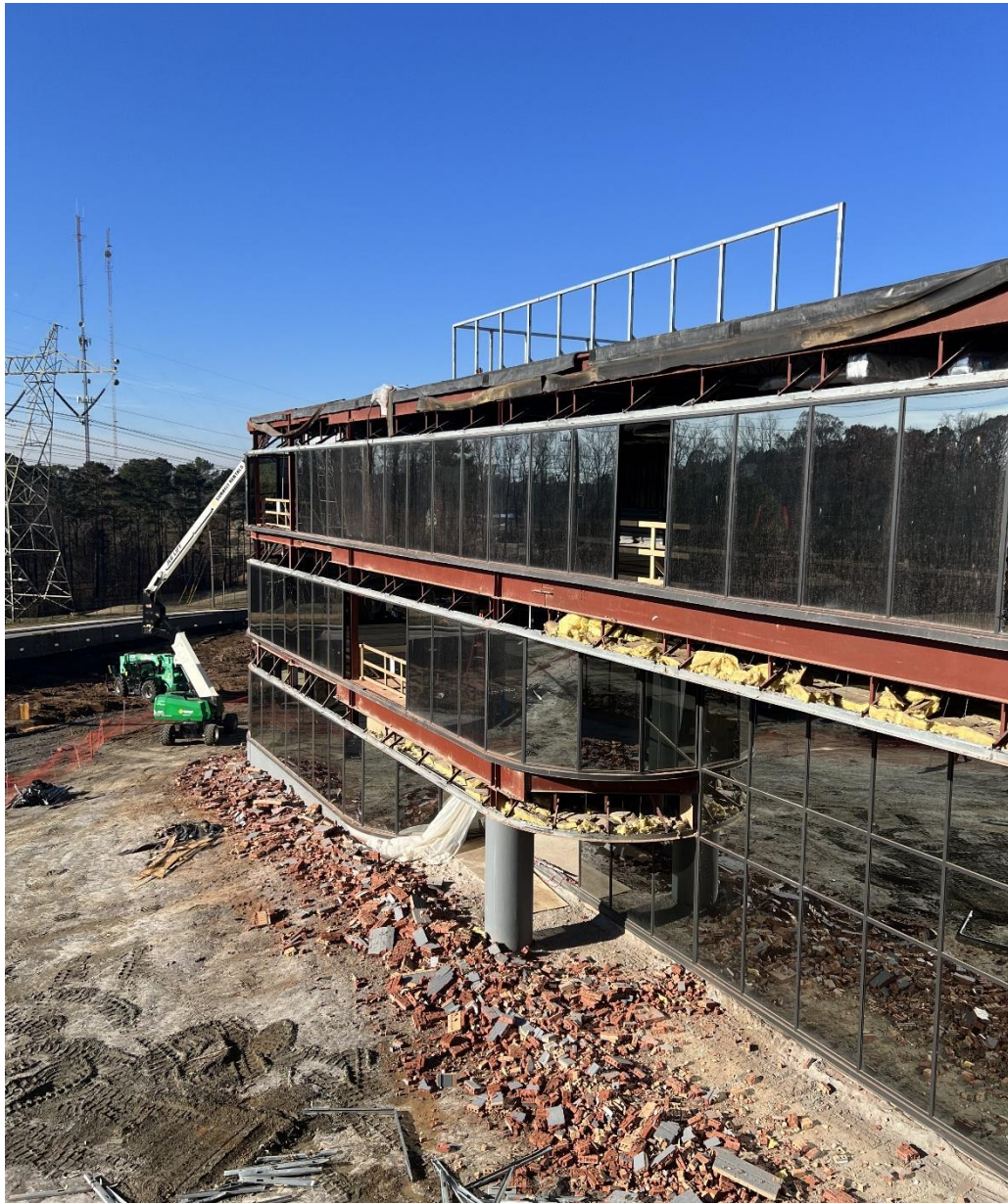
Continue Exterior Demo Brick/Glass/Lintel/Kicker - North Face
