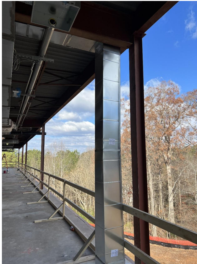
Mechanical Overhead Rough-in On Level 2
