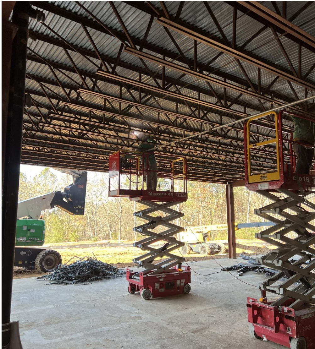
Joist Augmentation On Basement
