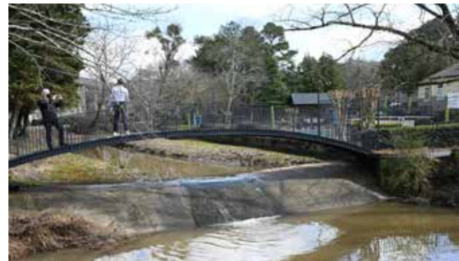
A dam/embankment across Long Island Creek
