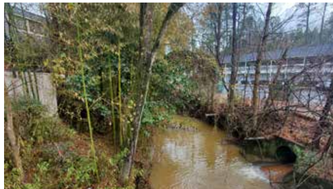
Stream bank conditions along Long Island Creek
