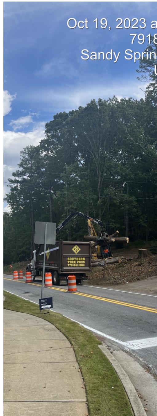
PW TS111 Temporary Striping
