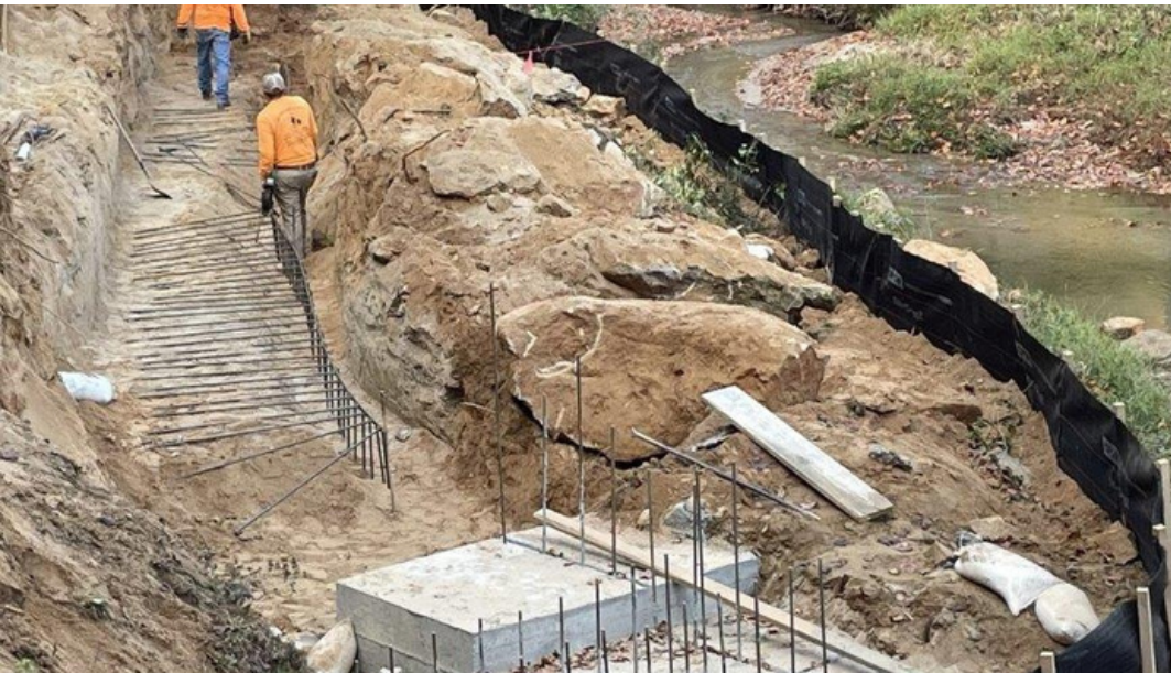
Springway Trail - Monterrey Bridge Footer Rebar
