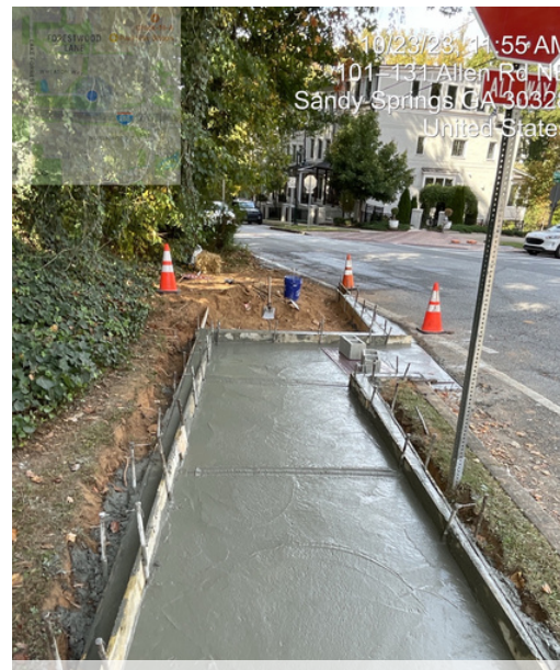
PW S2188-1 Sandy Springs Circle at Allen Road sidewalk ramp construction
