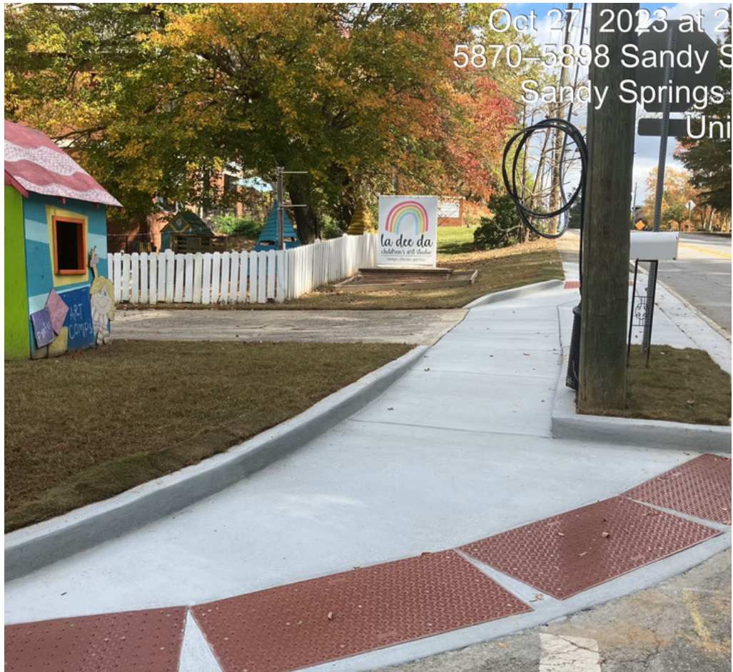
S2188 - Sandy Springs Circle at Allen Road -sidewalk construction
