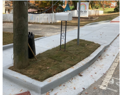
S2188 - Sandy Springs Circle at Allen Road -sidewalk construction
