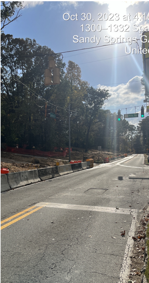
TS111 - Spalding Drive at Pitts Road - temporary roadway striping installed
