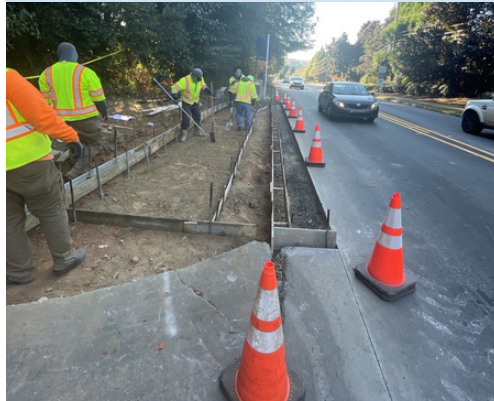
Springway Trail - working curb and gutter
