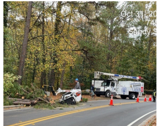
S2175 - Trowbridge sidewalk site clearing in advance of construction
