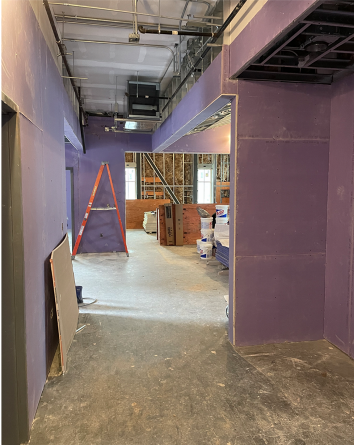
Continued Double-Siding on Second Floor with High Impact Sheetrock
