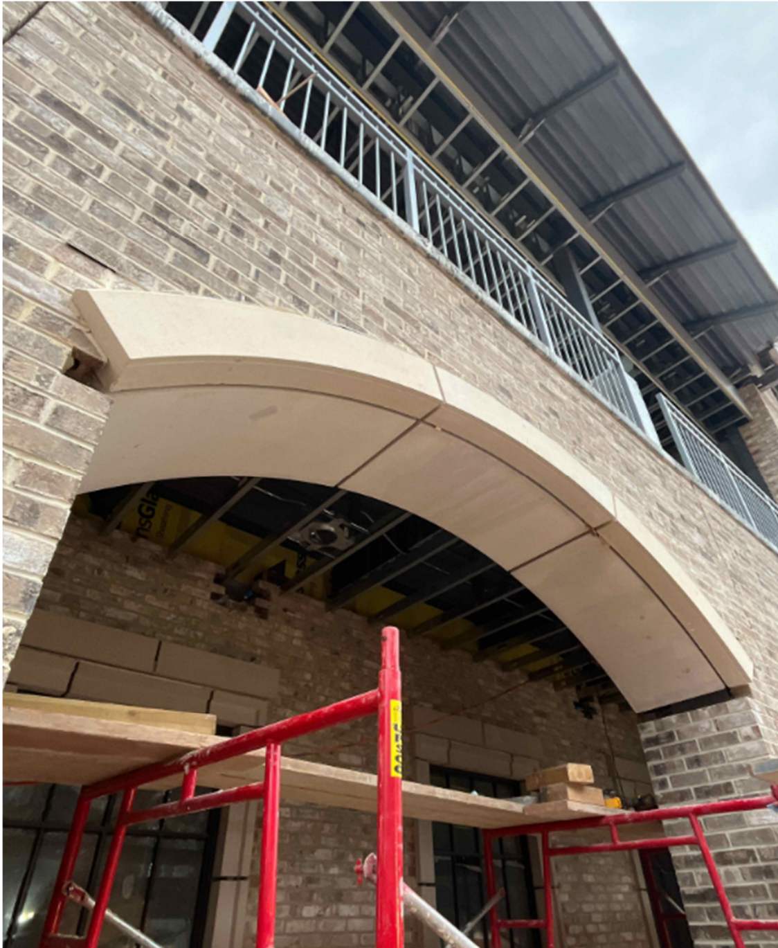
Continued Brick Veneer and Cast Stone Installation
