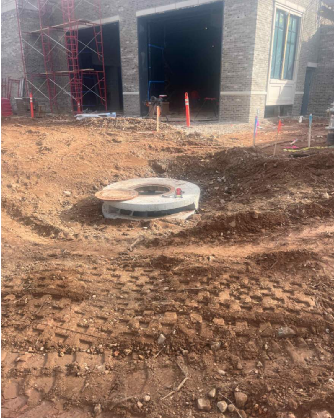
Installed Manhole Structures for Storm Line
