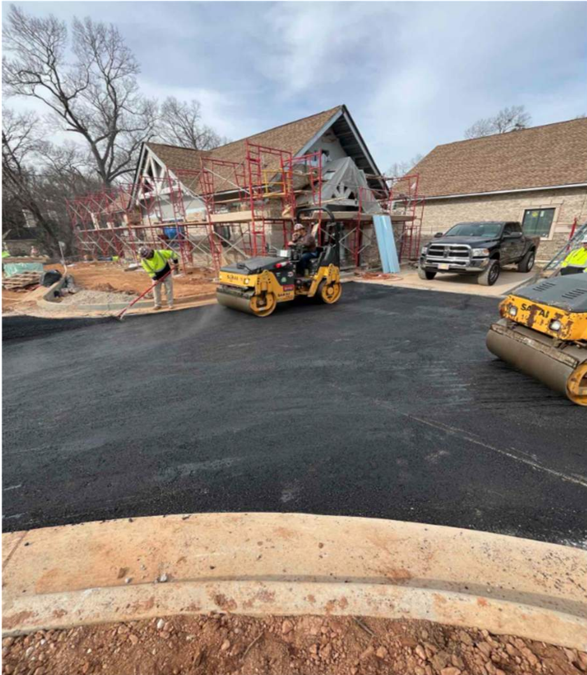
Poured Asphalt Paving at Mt Vernon Entrance
