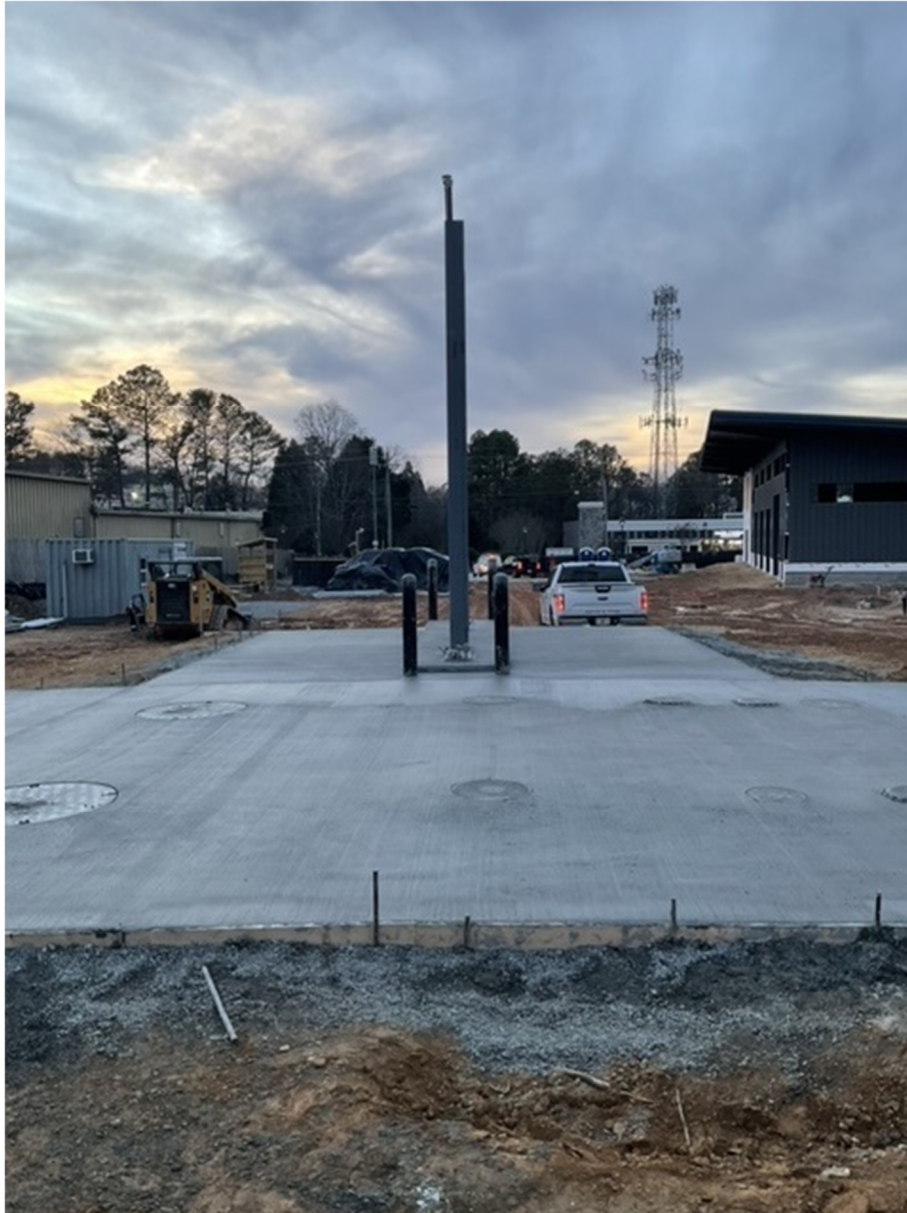
Poured Fuel Island & Pad
