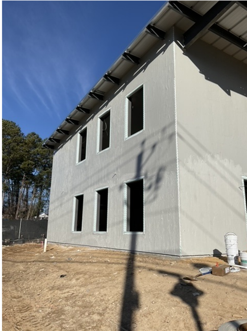
Applied Air Barrier
