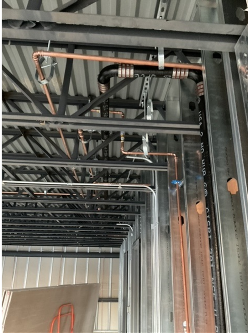
MEP In-Wall Rough-In
