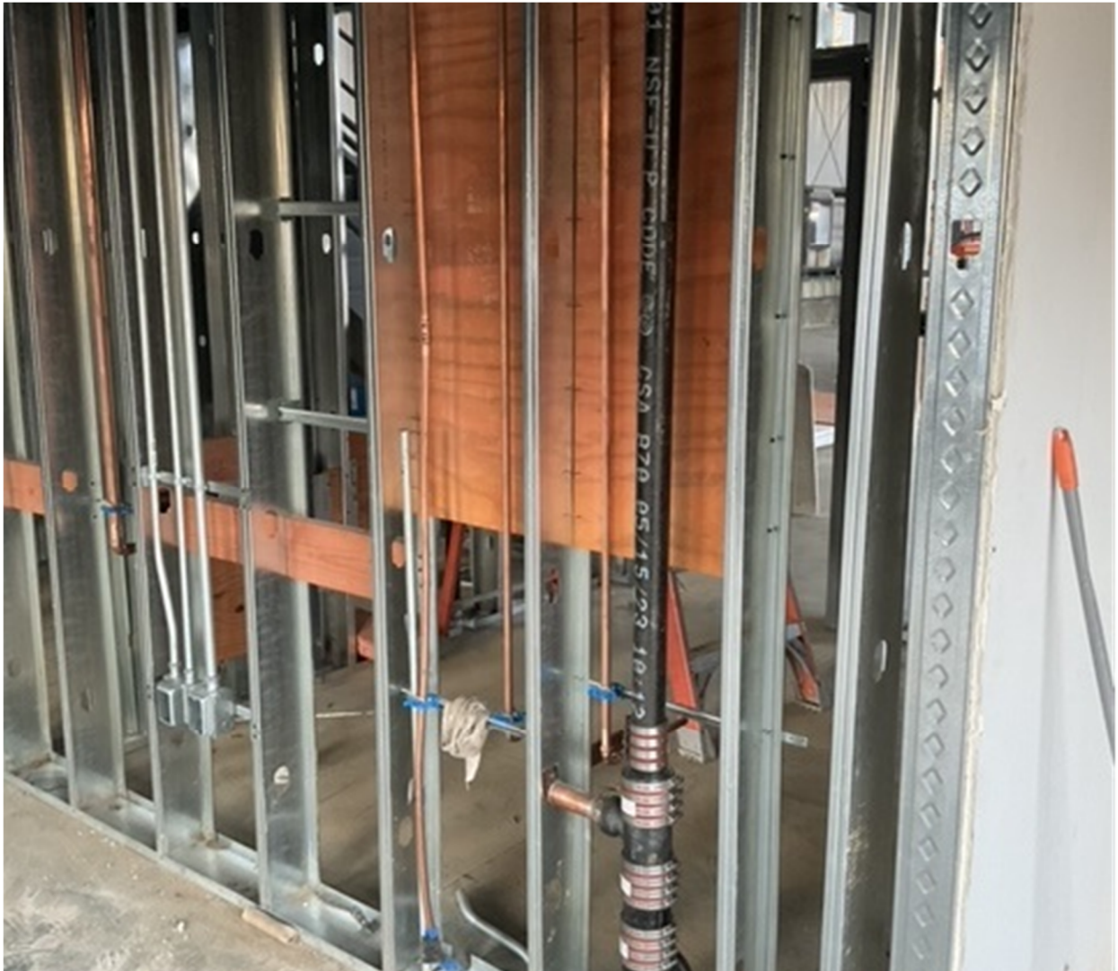
MEP In-Wall Rough-In
