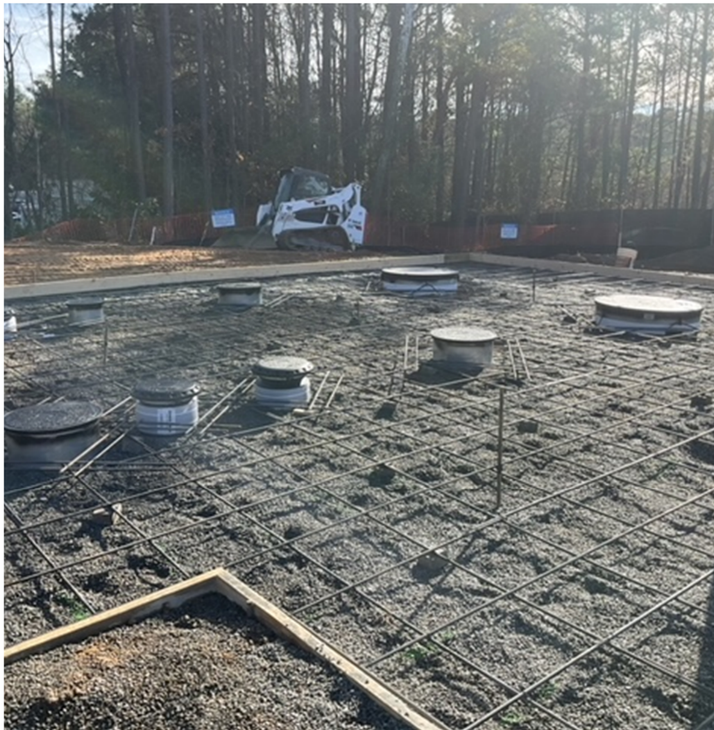
Rebar & Base at Fuel Island & Pad
