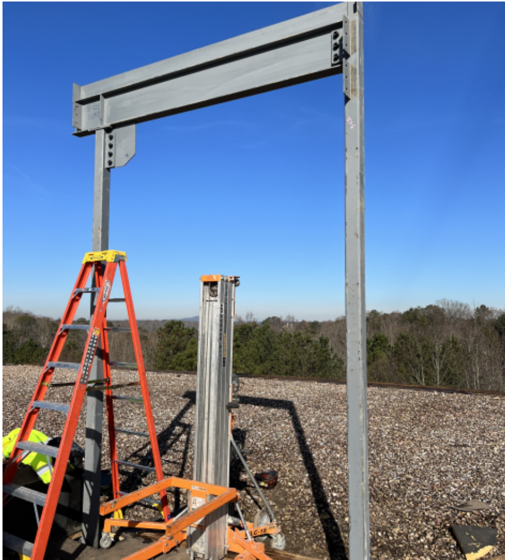
Steel for Roof Stairs
