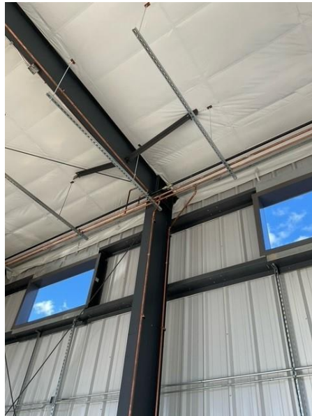
MEP Overhead & In-Wall Rough-In
