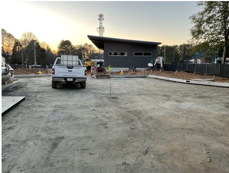
GAB Spread And Compacted In Back Lot
