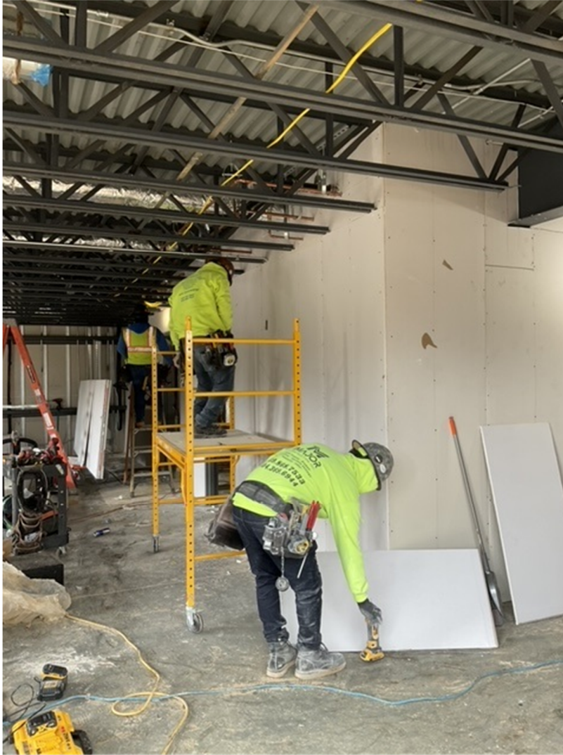
Sheetrock Installation
