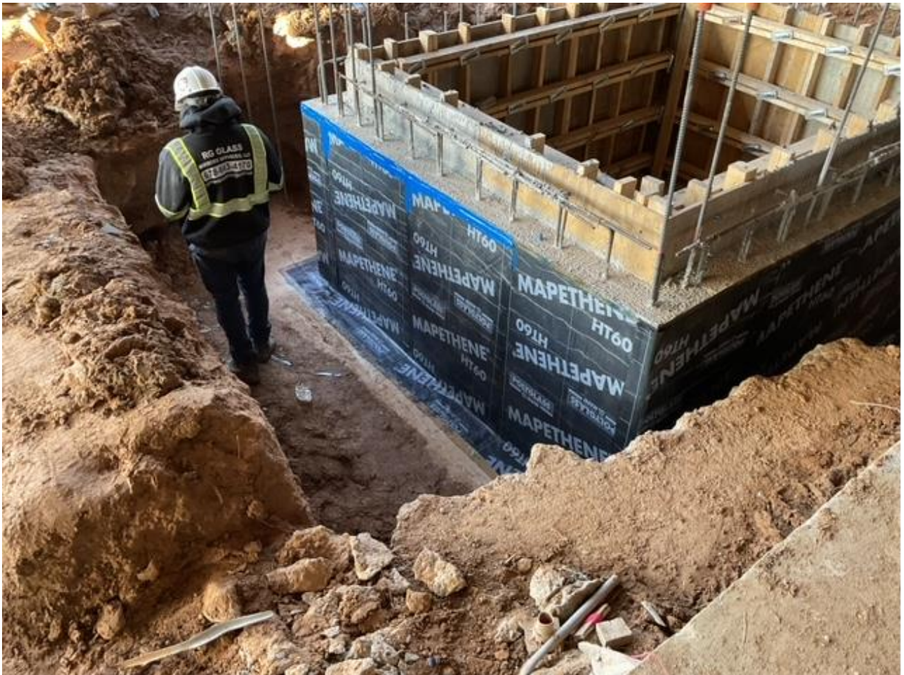
Waterproofing Elevator Pit Walls
