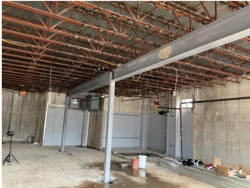
Setting Interior Columns/Beams at Basement
