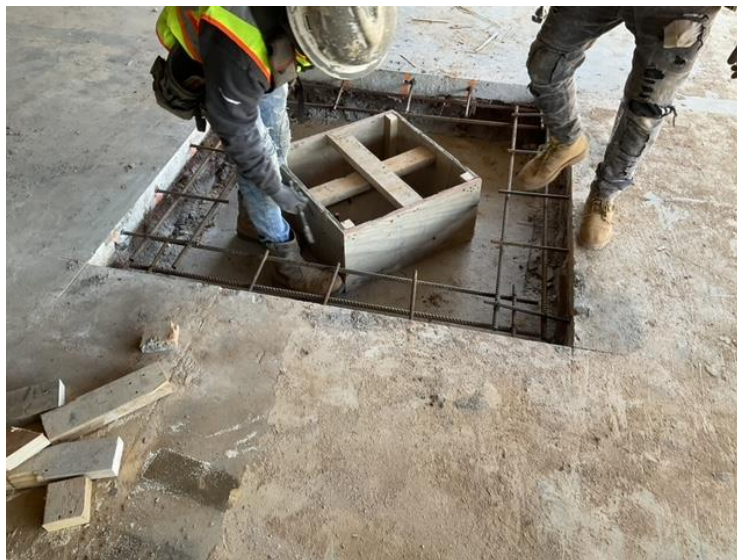
Concrete Work for Interior Columns
