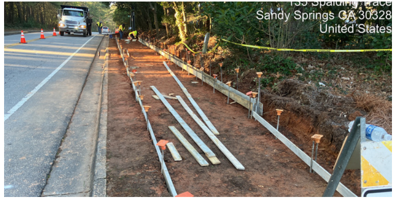
(TOP): S2188-3 GLENRIDGE SIDEWALK CONSTRUCTION (BOTTOM): TS108 - TRAFFIC CONTROL INSTALLATION
