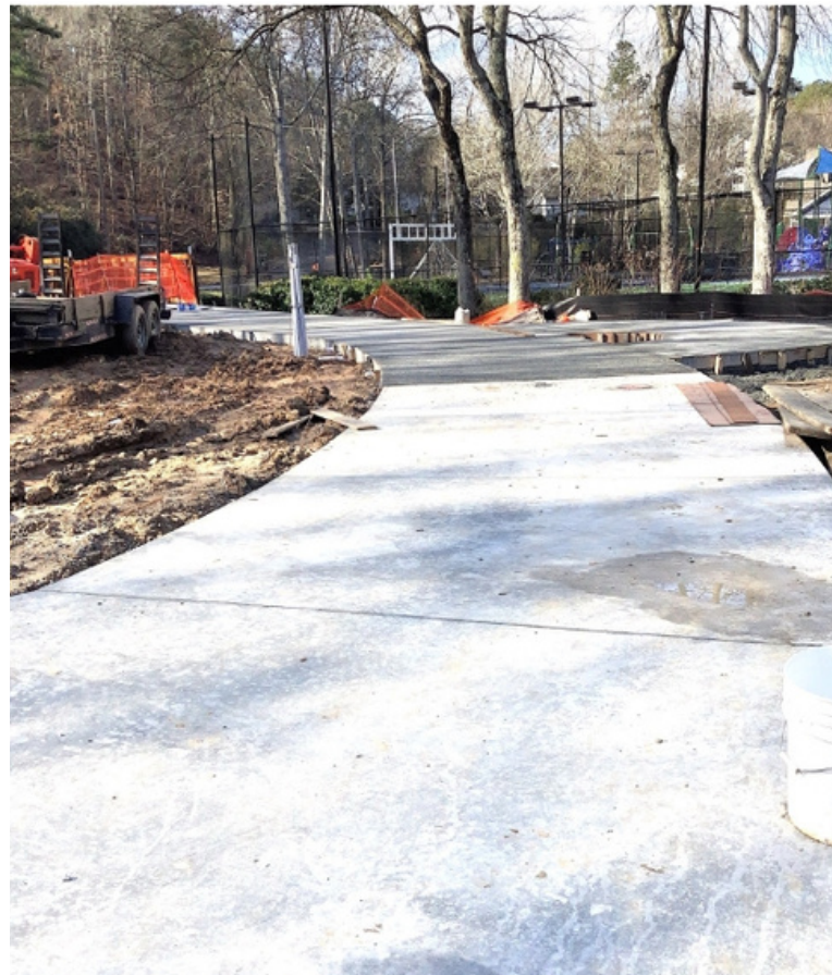
SPRINWAY TRAIL - MORE TRAIL POURED ON BOTH SIDES OF THE MONTEREY PARKWAY BRIDGE
