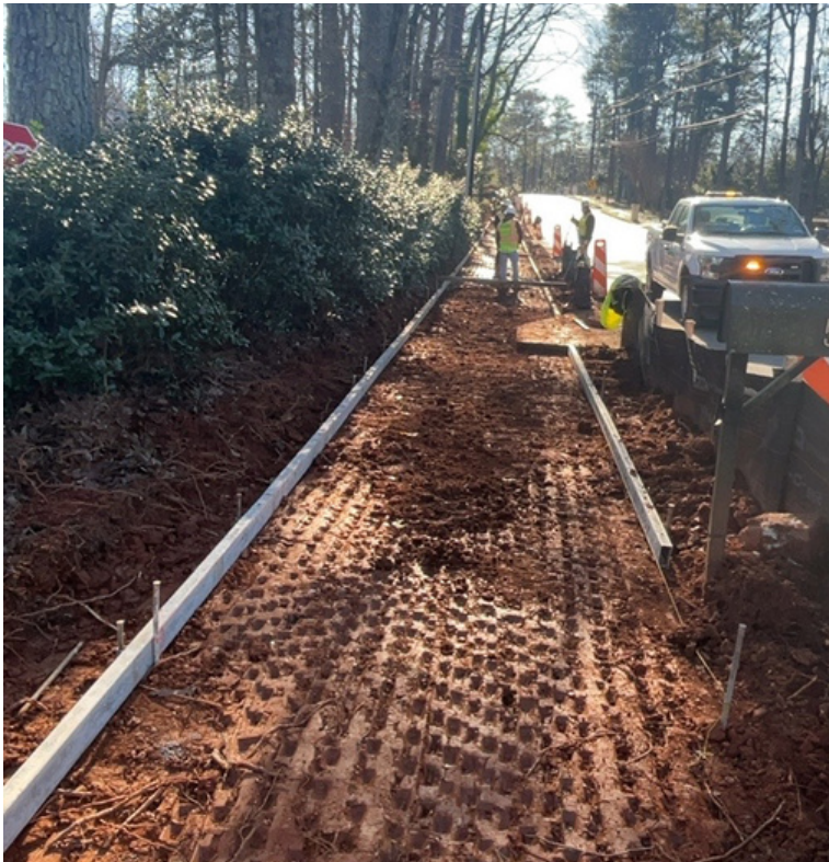
S2167 - MT VERNON SIDEWALK CONSTRUCTION
