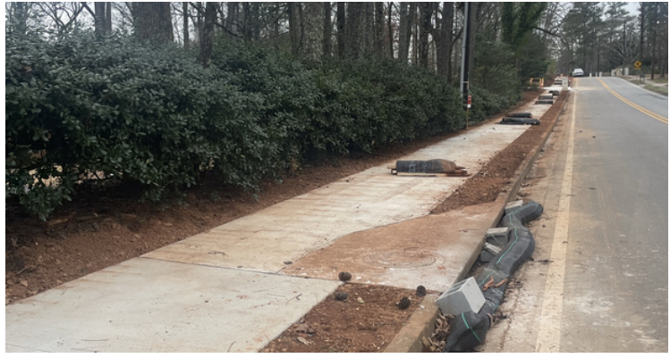
S2167 - MT VERNON SIDEWALK CONSTRUCTION
