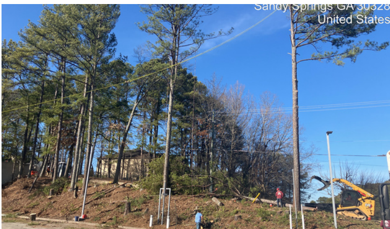
TS172 - GEORGIA POWER MOVING LINES TO NEW POLES
