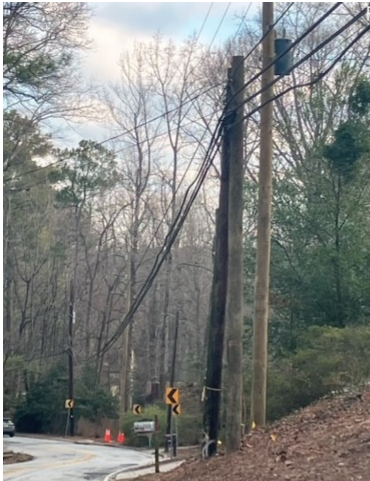
TS172 - GEORGIA POWER MOVING LINES TO NEW POLES
