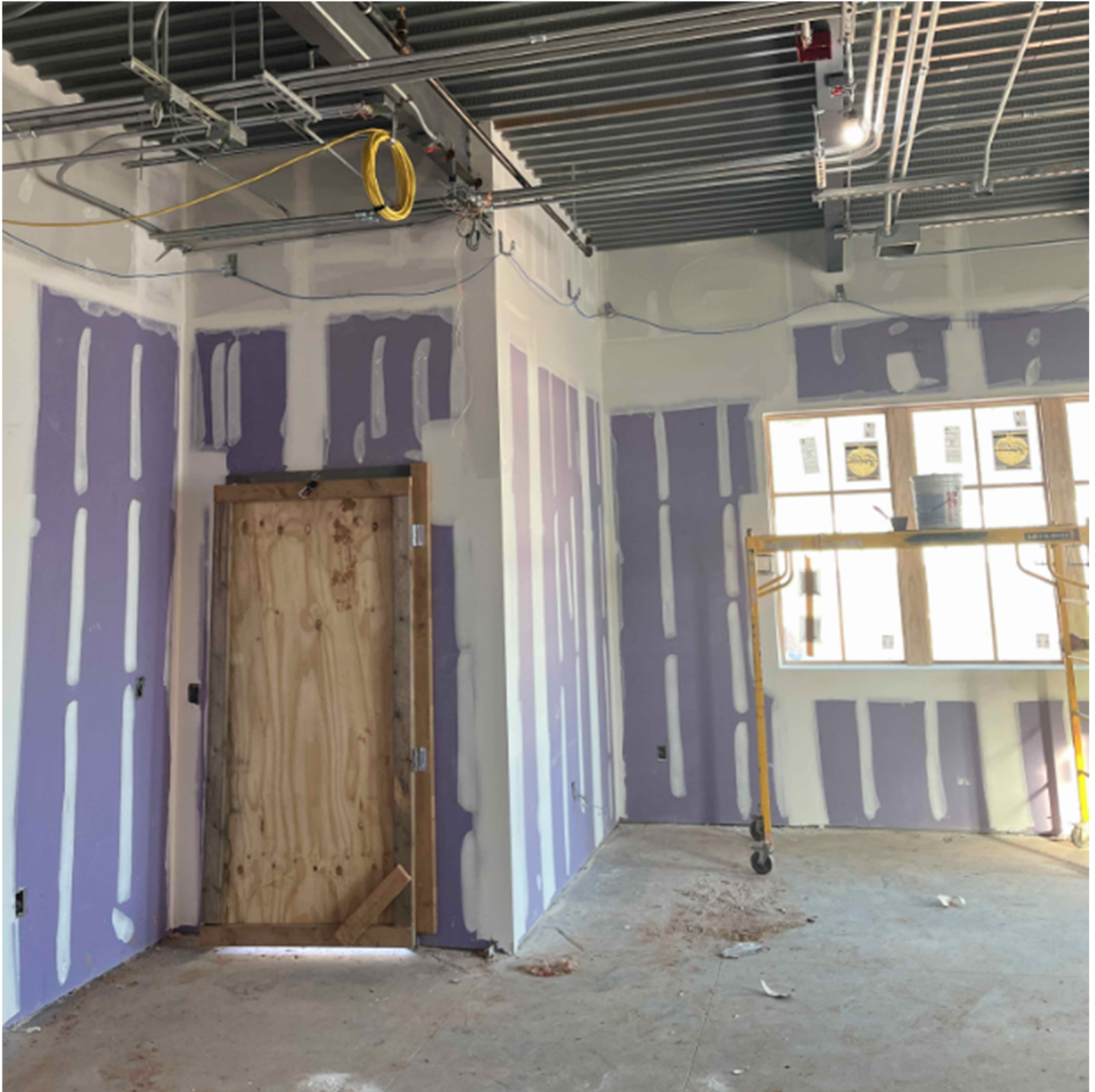
Began Mudding on First and Second Floor
