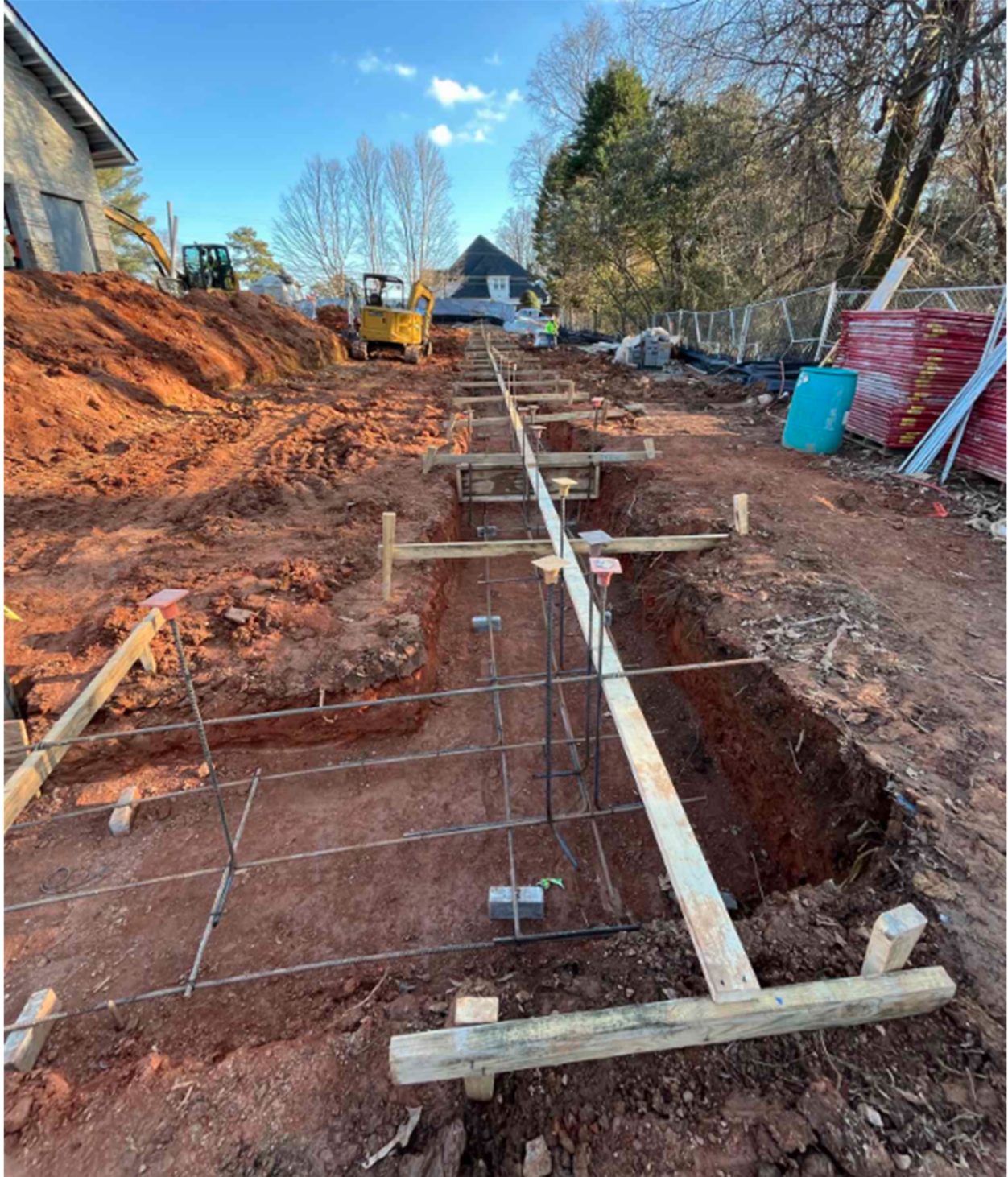
Began Prepping Screen Wall Footings
