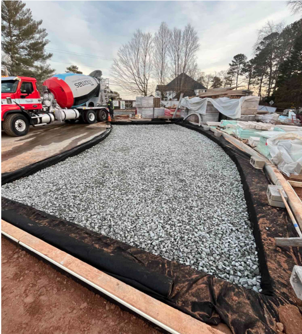
Began Prepping Parking Lot for Permeable Pavers
