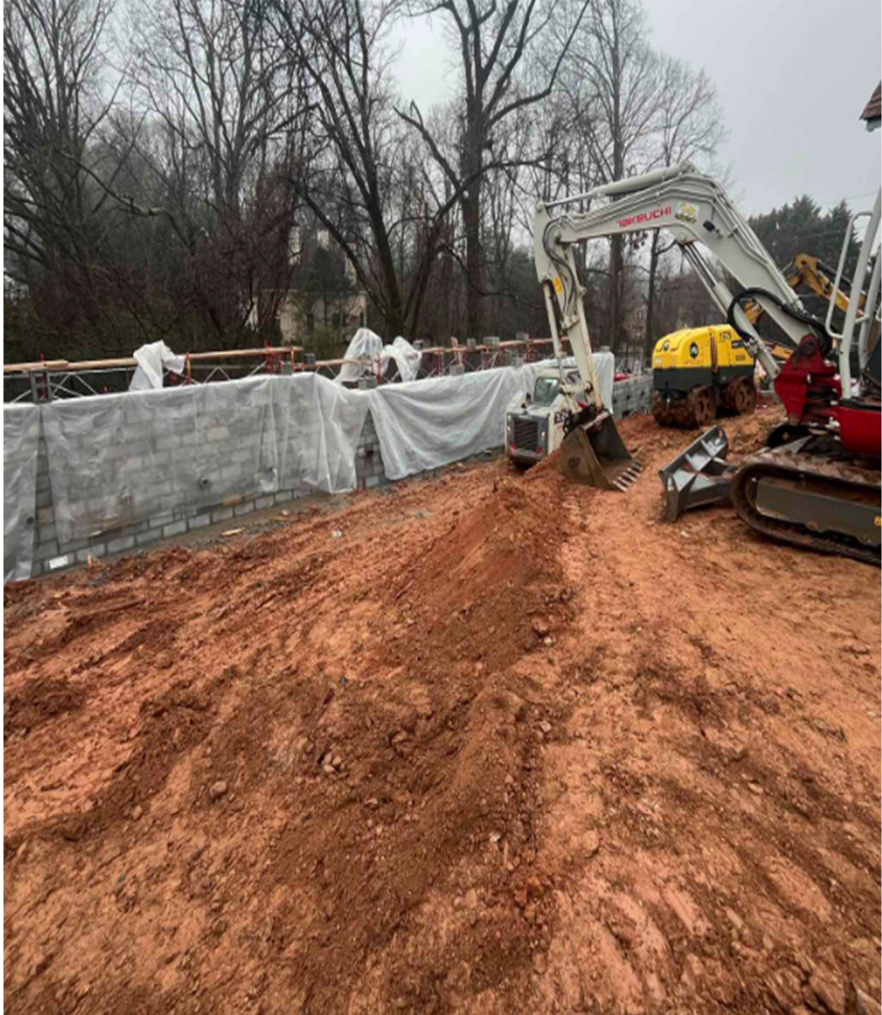
Began Screen Wall Blocking
