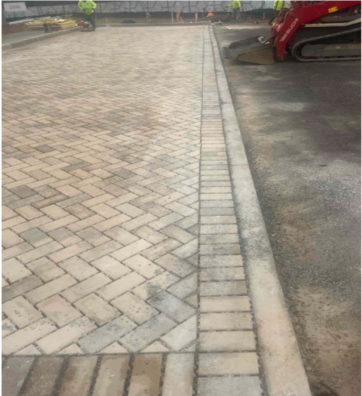
Began Laying Permeable Pavers at Mt Vernon Entrance
