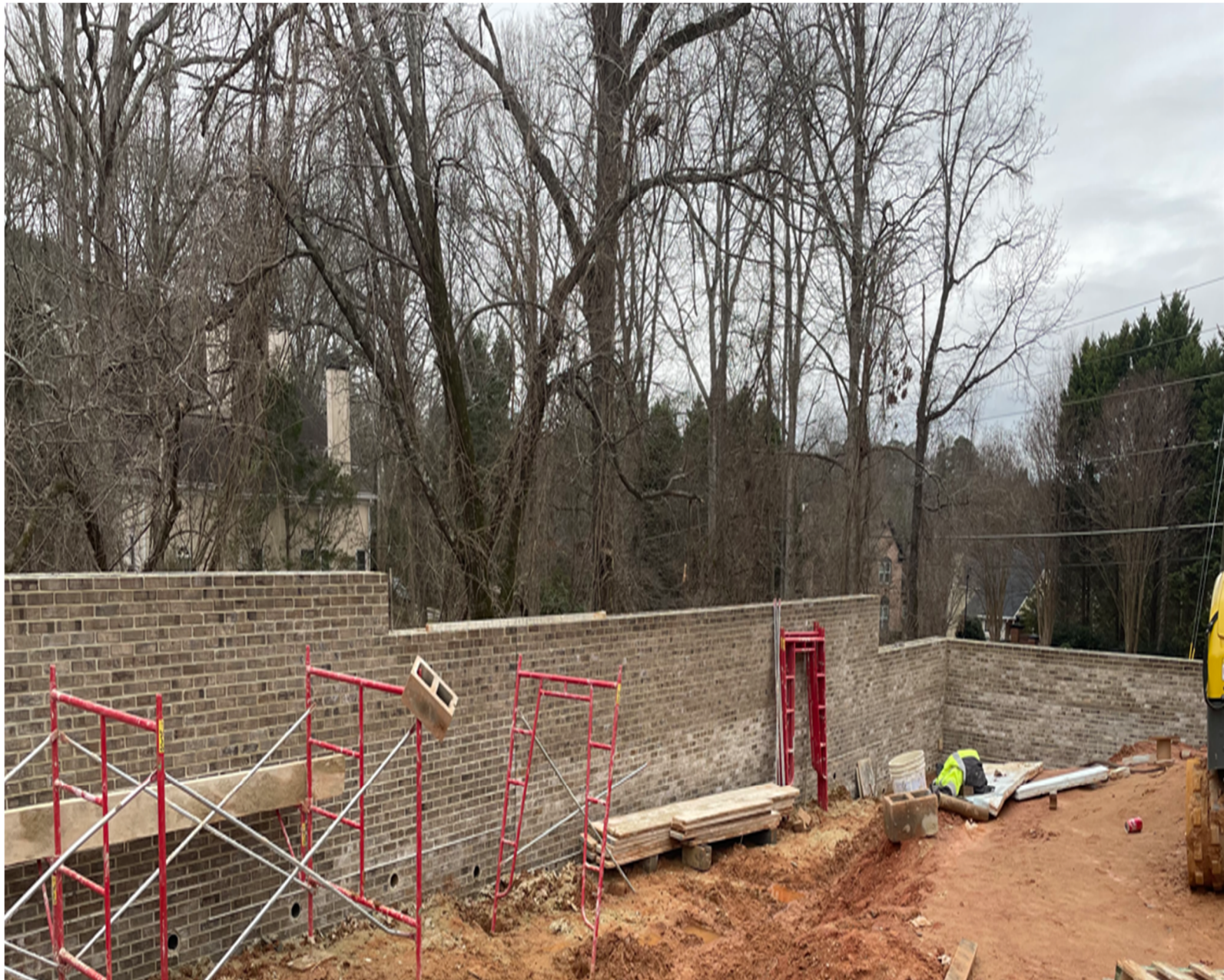
Continued Screen Wall Installation
