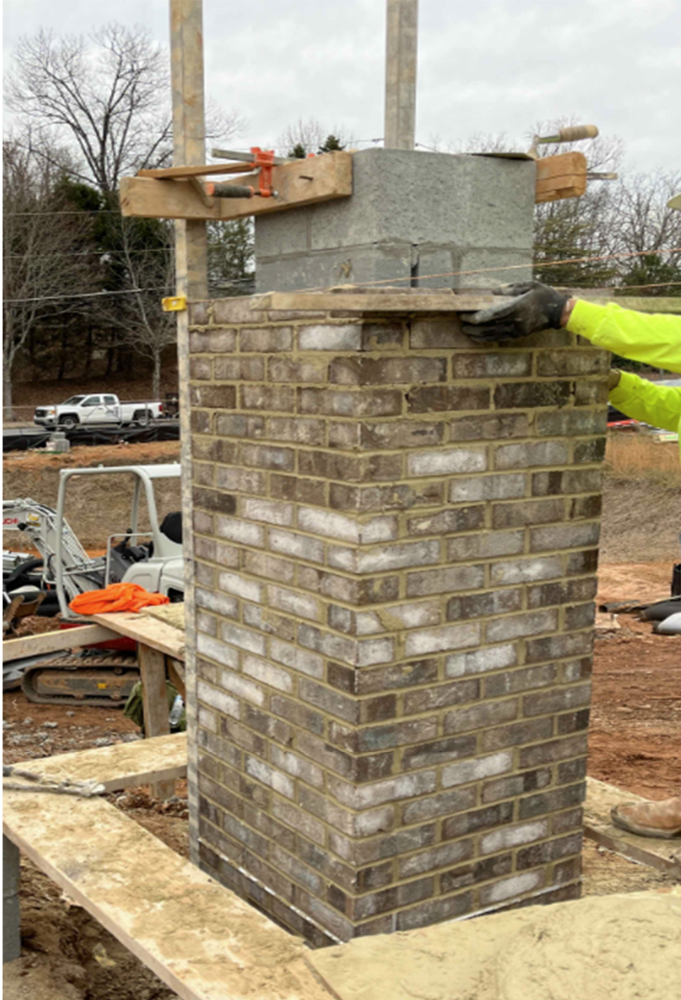
Began Installing Brick Veneer and Cast Stone Pillars for Site Fencing
