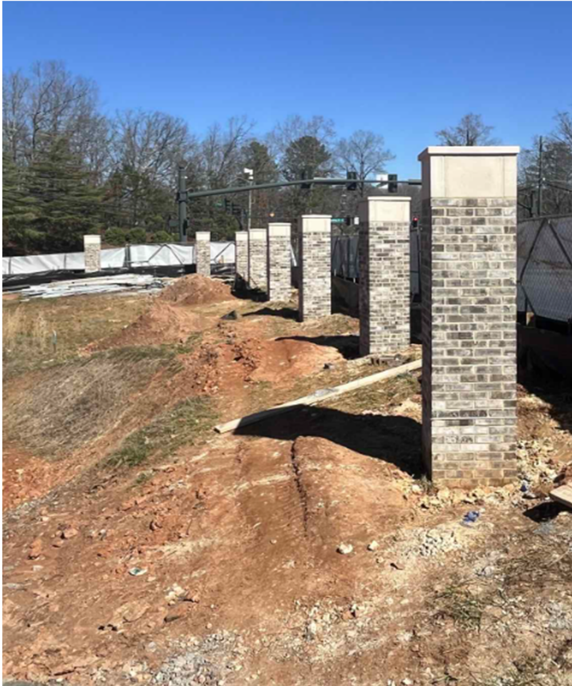
Continued Installing Brick Veneer and Cast Stone Pillars for Site Fence
