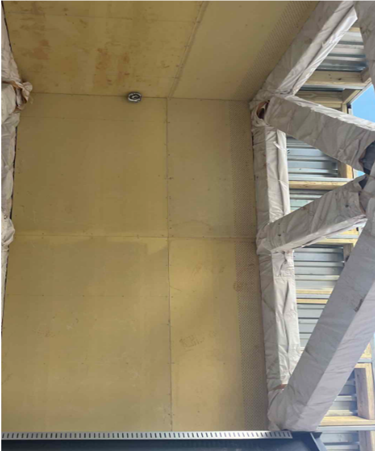
Began Installing Fiber Cement Soffit and Siding
