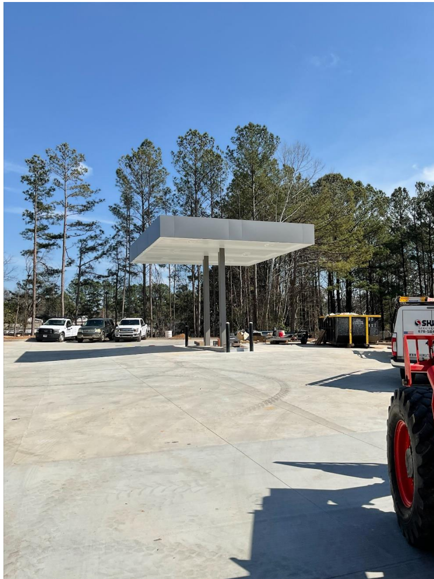
Fuel Canopy Was Completed
