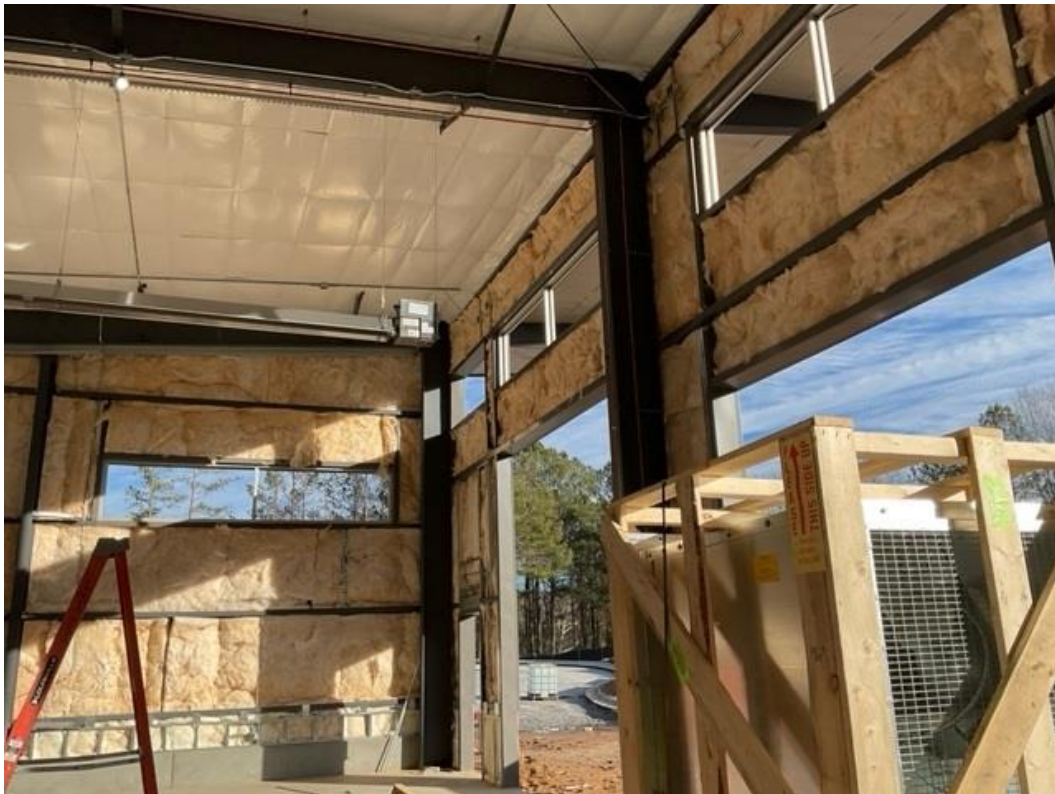
Building Insulation Was Installed
