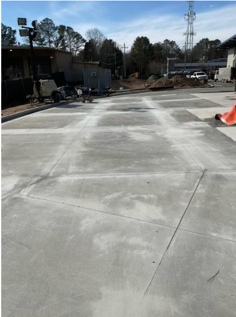
Sawcut Control Joints In The Parking Lot
