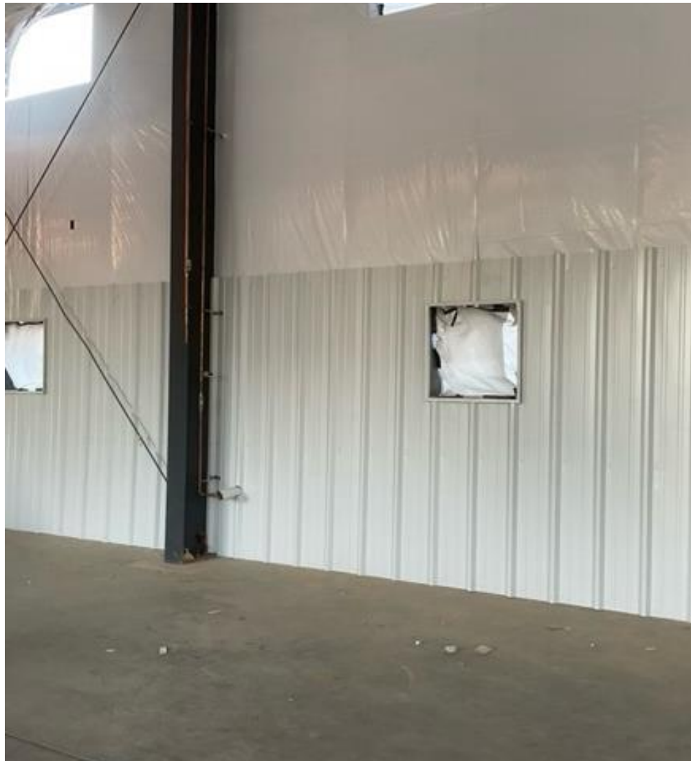
Interior Metal Panels Were Installed
