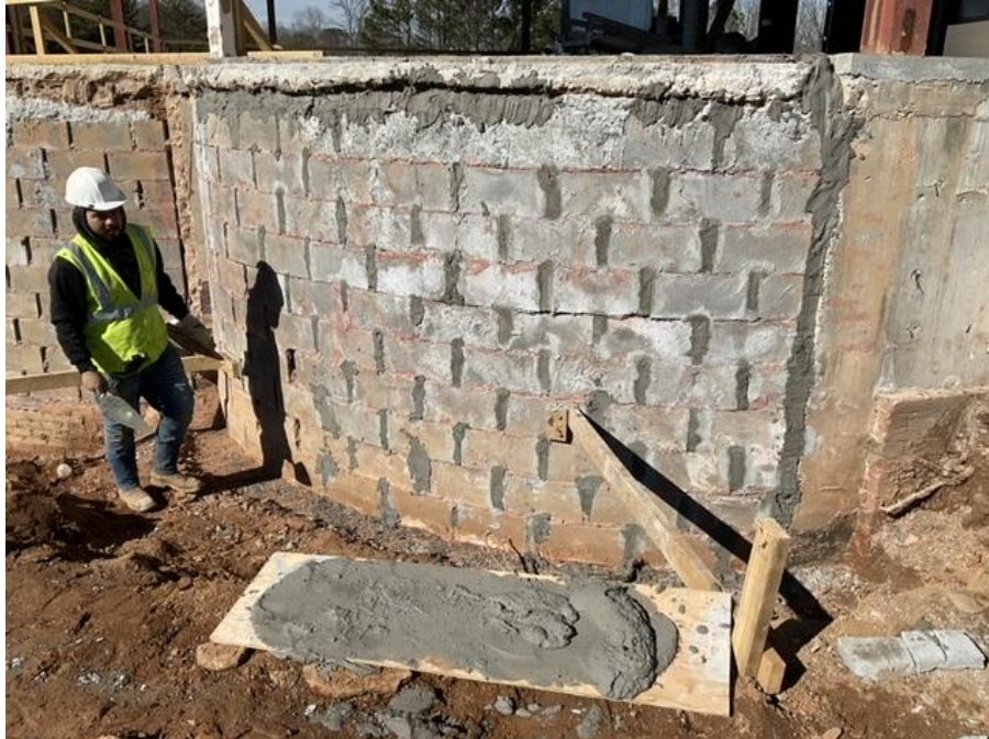
CMU Wall Remediation
