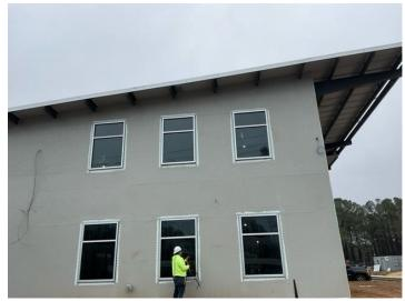
Glass Installed In Window Frames
