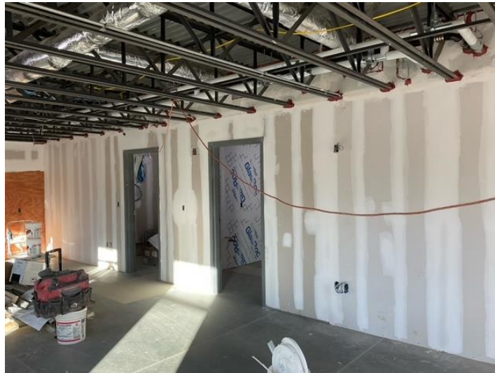
Began Drywall Finishing
