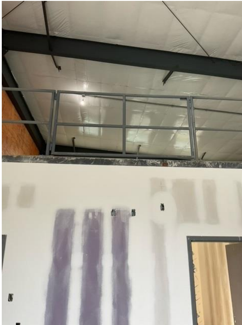
Mezzanine Gate Installed
