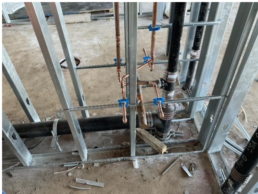
In Wall Plumbing Rough-In
