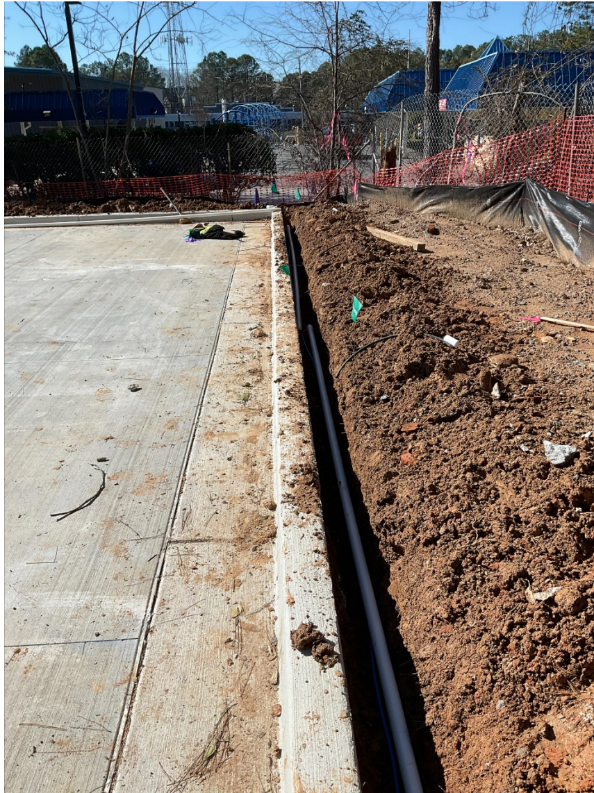
Began Running Irrigation
