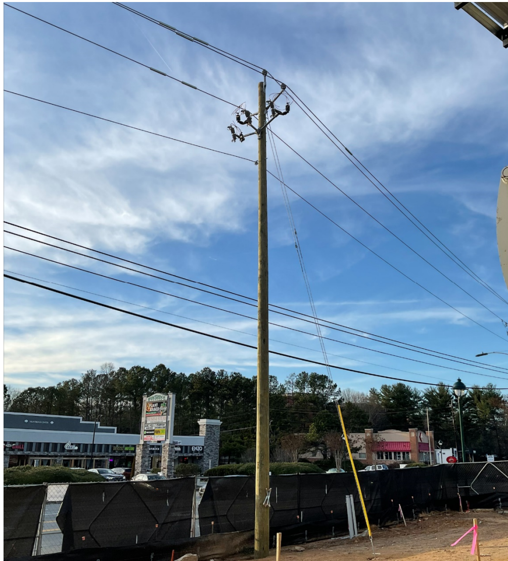
New Power Pole Installed (GA Power)
