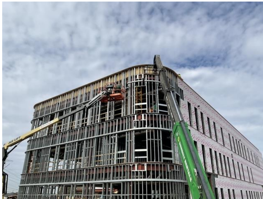
Brick Lintel Installation (North Elevation)
