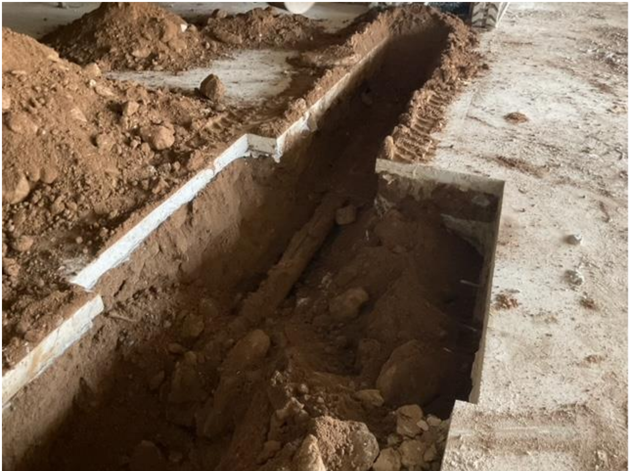
Replacement Of U/G Sanitary Sewer Piping - Basement
