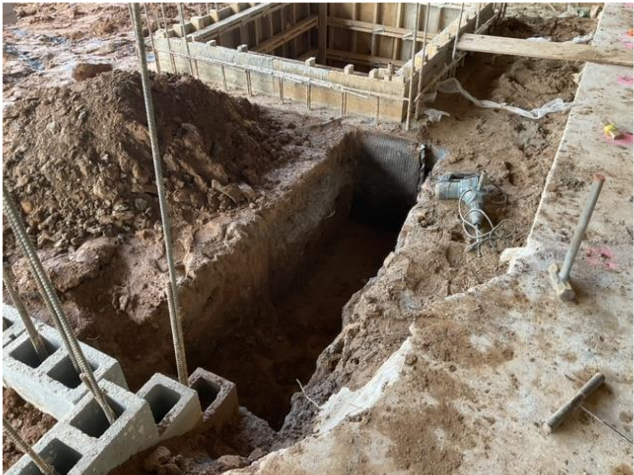
Footings At Holding Cell & Elevator Areas
