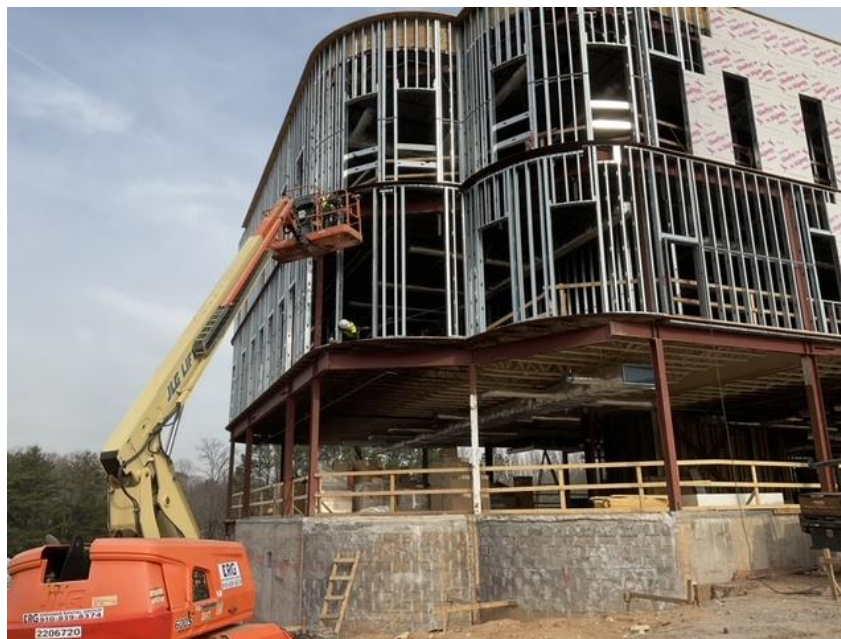
Exterior Framing/Sheathing Southwest Elevation
