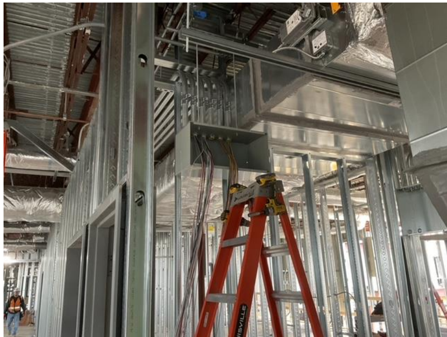
O/H & In Wall Electrical Rough-In - Level 3
