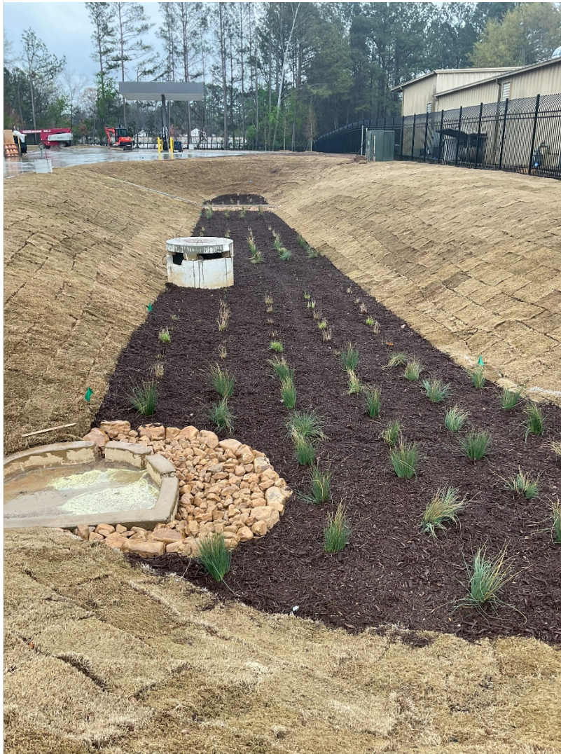
Bio-cell Pond Completed
