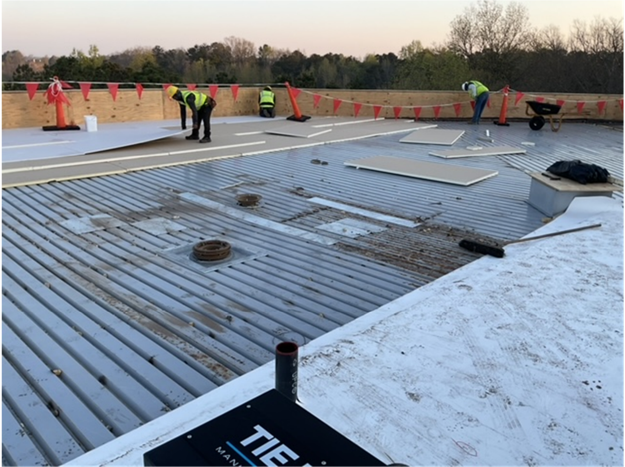
New Roof Install
