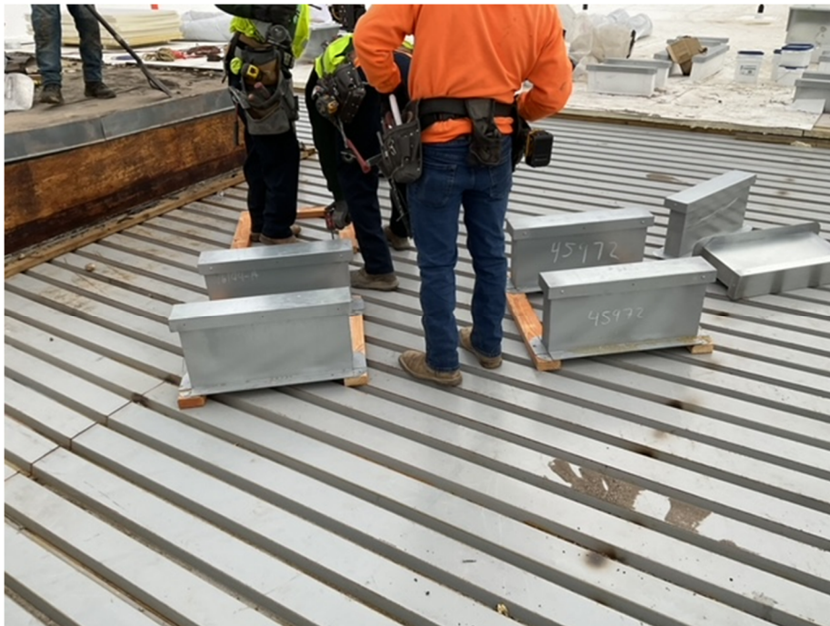
New Roof Install
