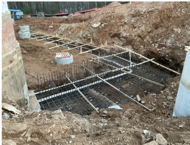
Rebar Formwork For Retaining Wall B
